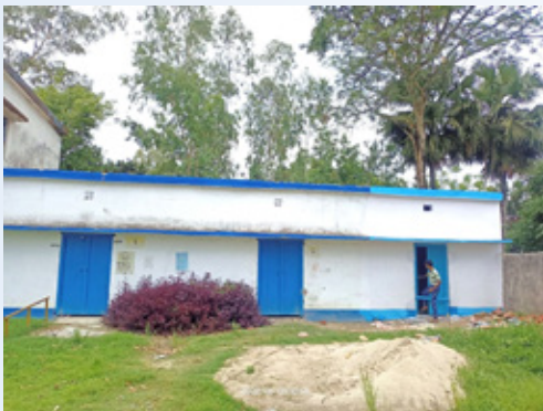
Completed additional room construction by MSTC at Jidhra Primary School, South Dinajpur, W.B. under CSR
