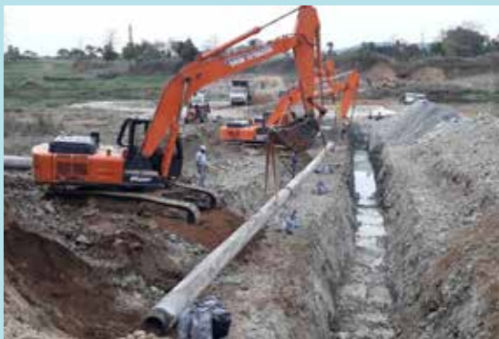
Cross-Country Pipeline Projects (CCP)
