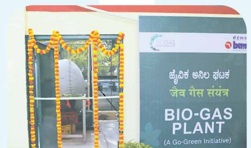
New Bio Gas Plant at Bangalore Complex towards Go-Green Initiative.
