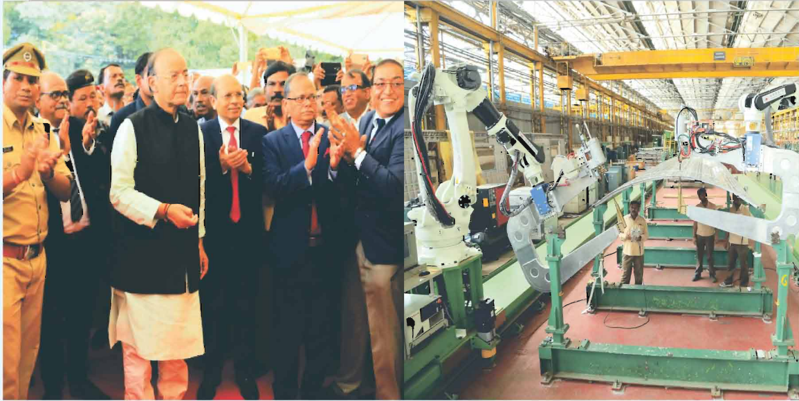
Shri Arun Jaitley Hon'ble Finance Minister and the then Hon'ble Defence Minister inaugurating 3 rd line Metro facility at Bengaluru Complex in the presence of Shri Deepak Kumar Hota, CMD BEML. The new hangar will enhance increase metro car production.
