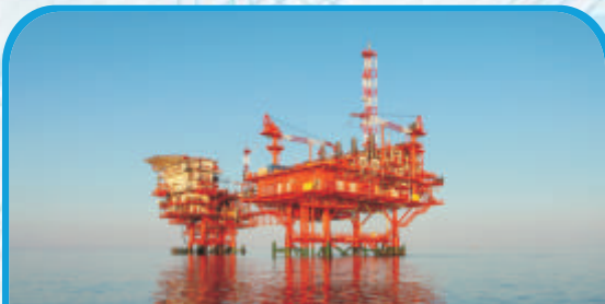
Oil & Gas, Petrochemicals & Chemicals
