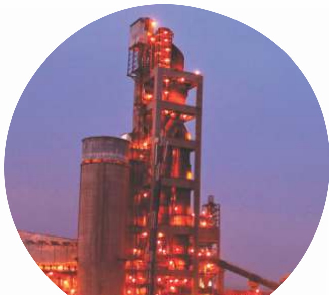
INTEGRATED CEMENT UNIT AT DURG
