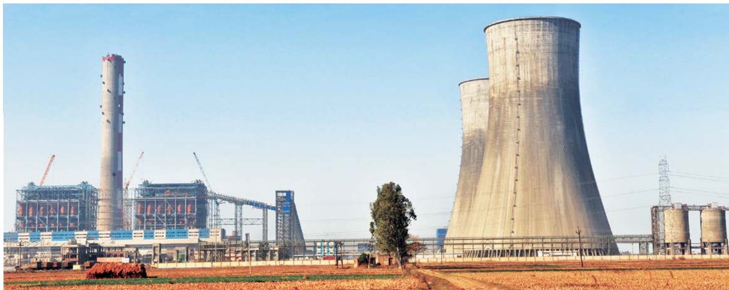
Rajpura project at the cusp of completion in December 2013
