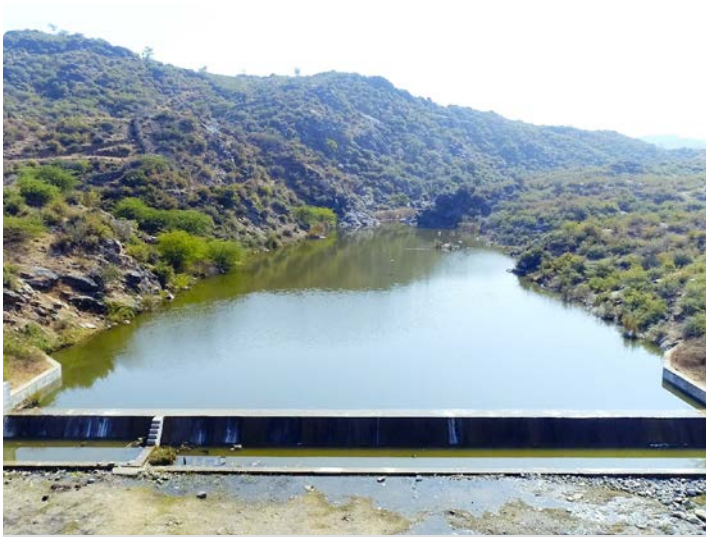
L&T has built over 200 check-dams in rural water-stressed areas
