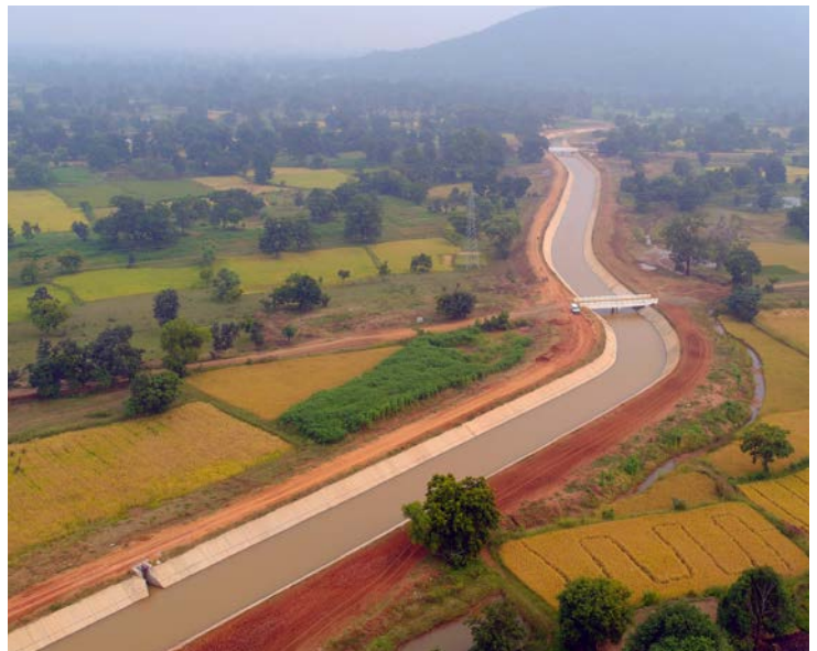
Lift Canal System for Upper Indravati Irrigation Project, Odisha
