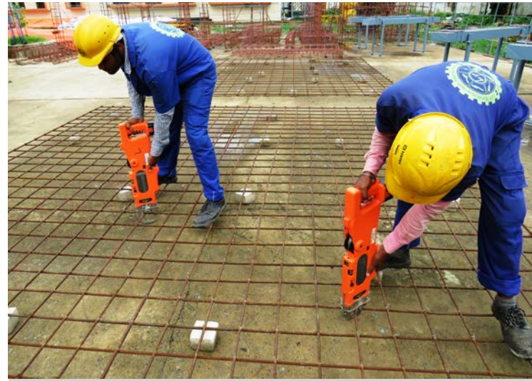
Training with bar-tying machine at one of L&T's CSTIs
