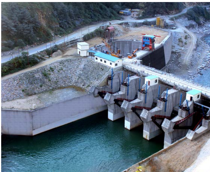
Singoli Bhatwari Hydro Power Project, Uttarakhand
