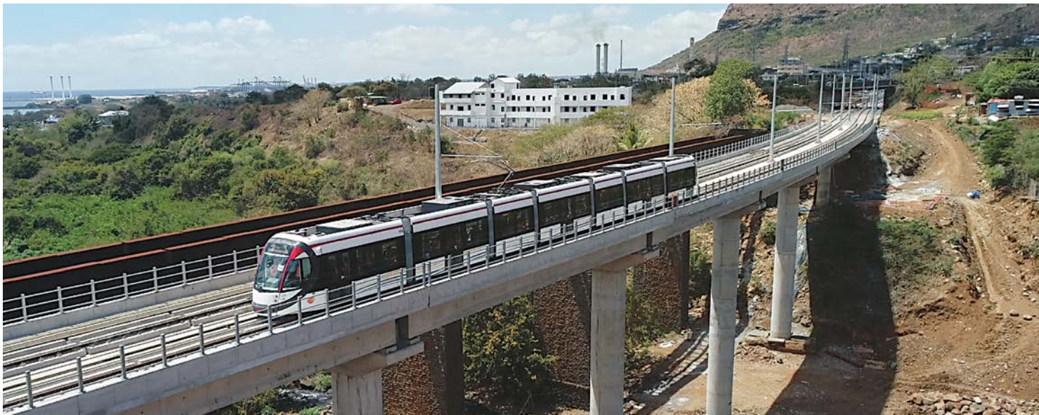
A section of the 13km Phase 1 of Mauritius Metro
