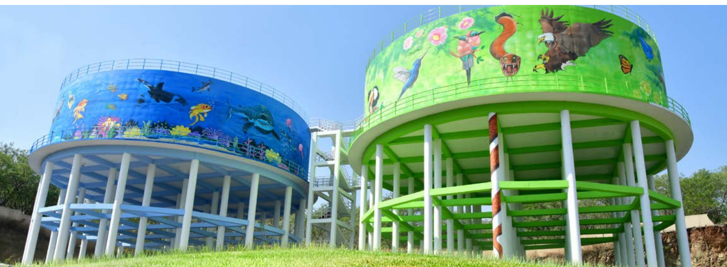
Elevated Storage Reservoirs at Pune, Maharashtra
