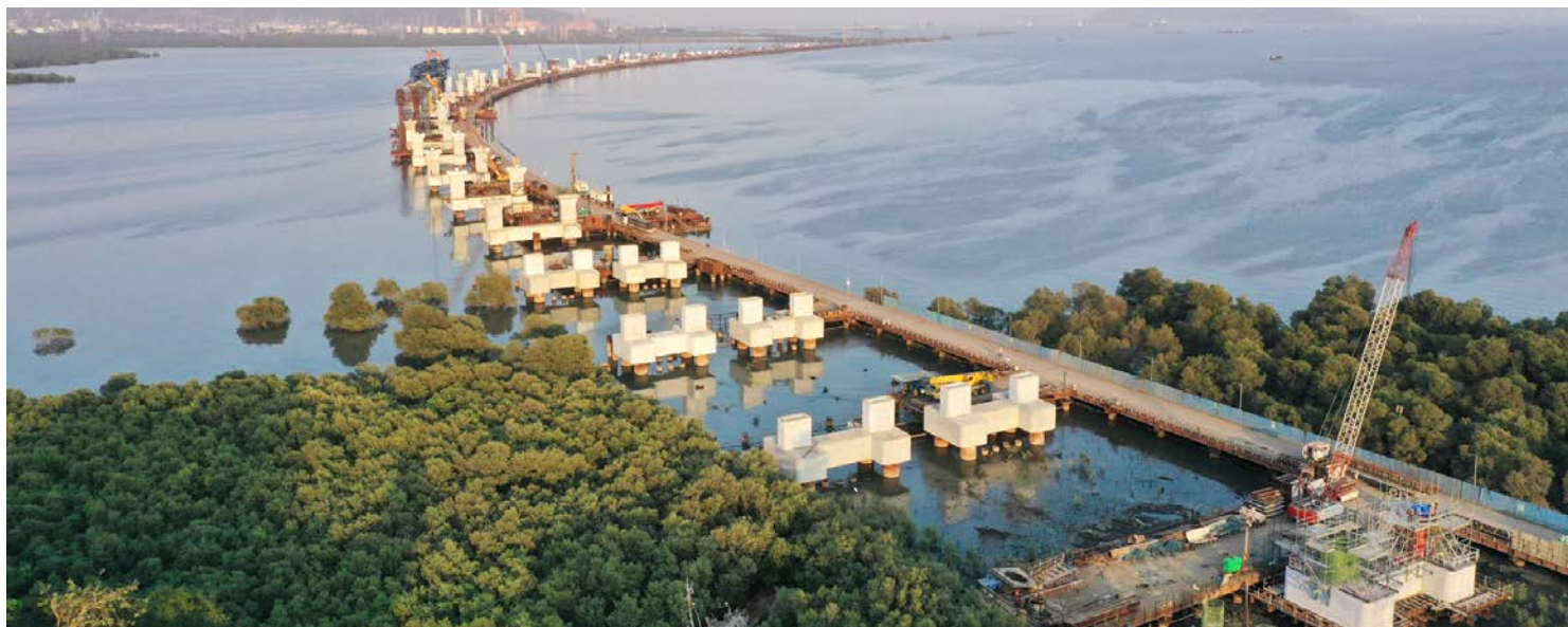
The Mumbai Trans Harbour Link
