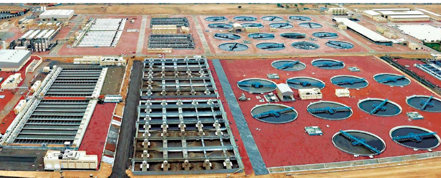
375 MLD Sewage Treatment Plant, Jebel Ali, UAE
