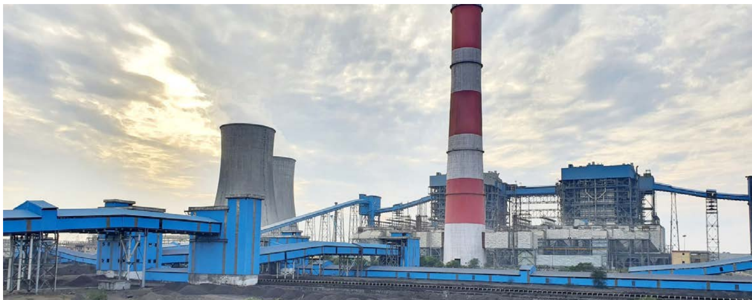
Chhabra Coal Handling Plant, Rajasthan
