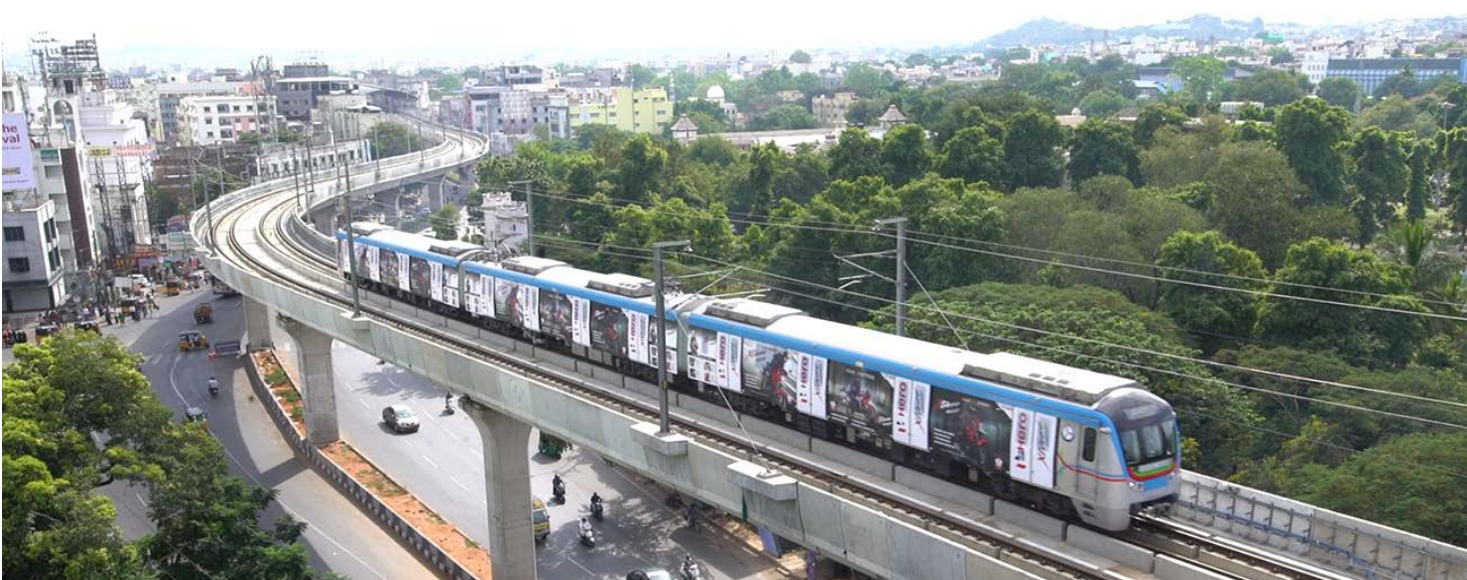
Hyderabad Metro Rail on the Viaduct
