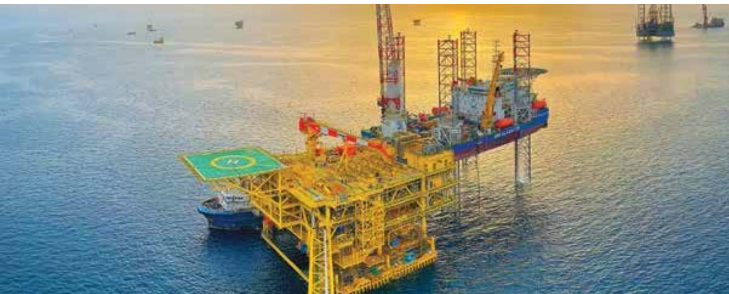
The heaviest fully integrated gas platform in Saudi Aramco's history installed by float-over method at the Hasbah field in Saudi Arabia
