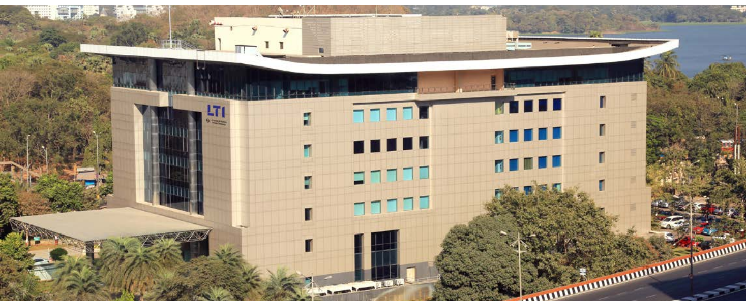
LTI Headquarters, Powai, Mumbai
