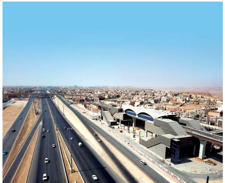
Riyadh Metro Line 3, Kingdom of Saudi Arabia
