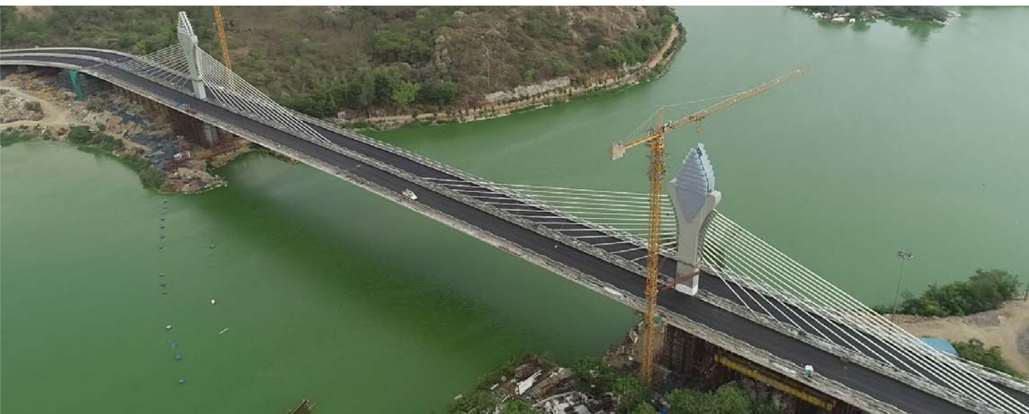
Cable Stayed Bridge across Durgam Cheruvu Lake, Telangana
