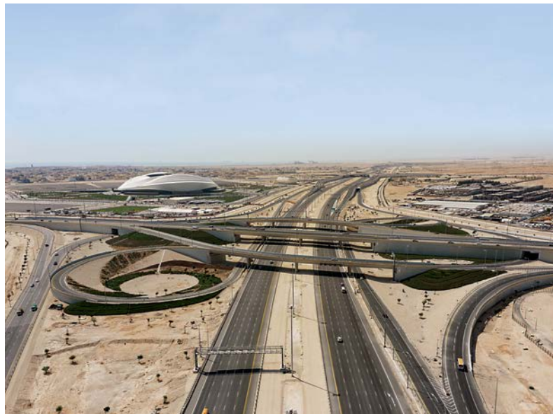
Al Wakrah Bypass Road Project, Qatar
