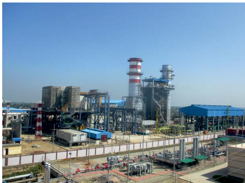
400 MW Combined Cycle Power Plant, Bibiyana-III, Bangladesh
