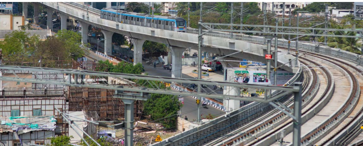
Sharp bend of the Viaduct
