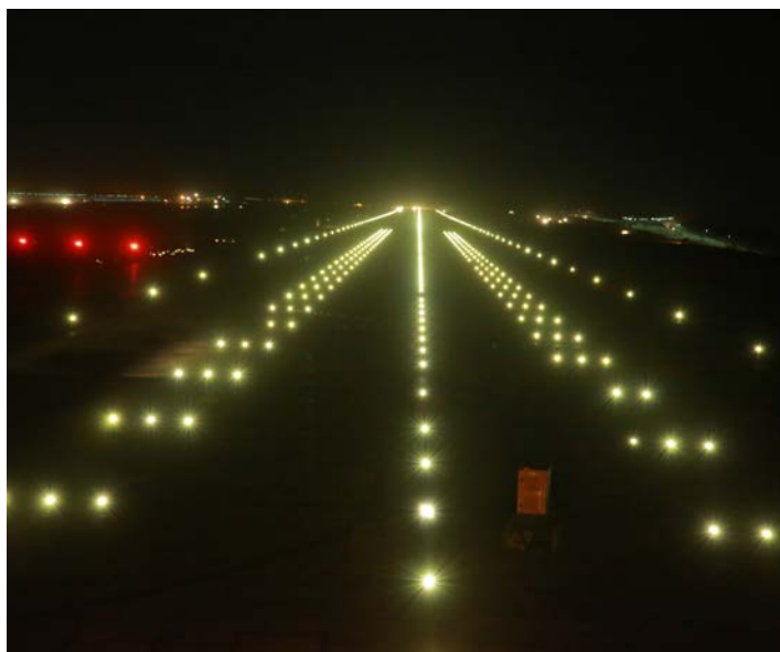
Runway for Bengaluru International Airport
