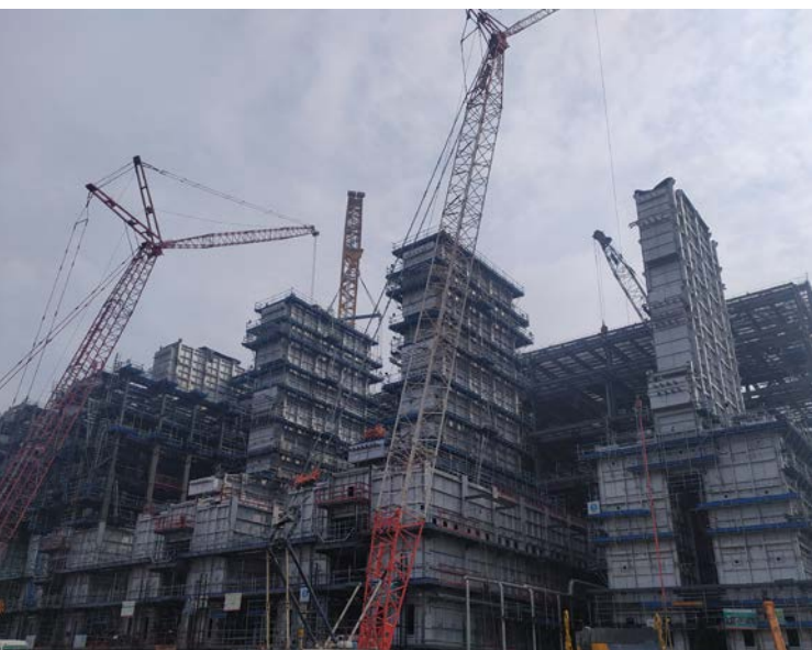
Cracker Furnace Package under execution for HMEL, Bathinda, India
