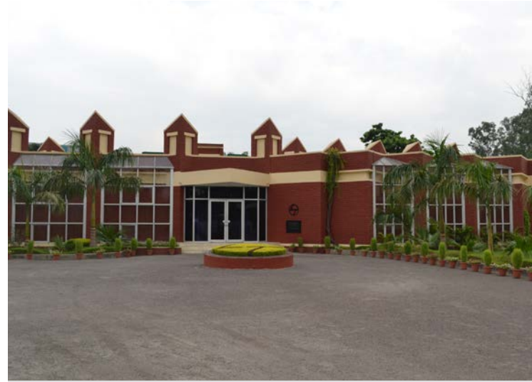
L&T's Switchgear Training Centres promote good electrical practices
