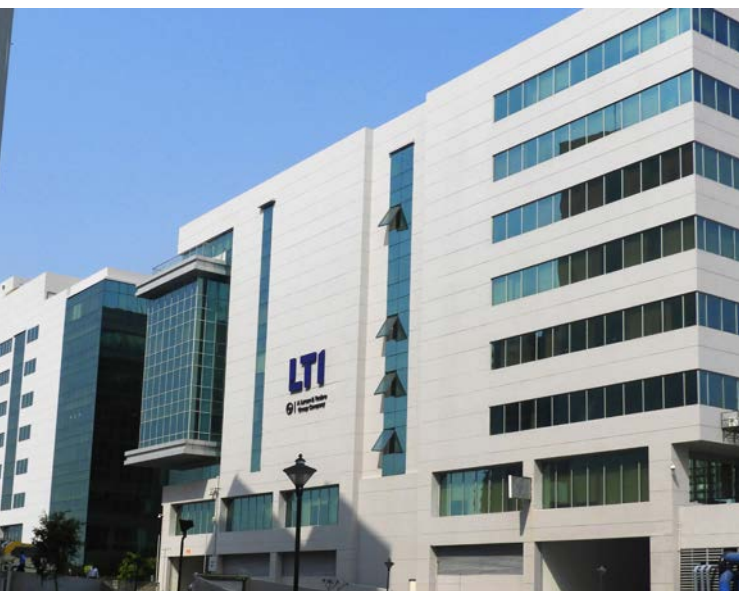
LTI's Delivery Center at Pune
