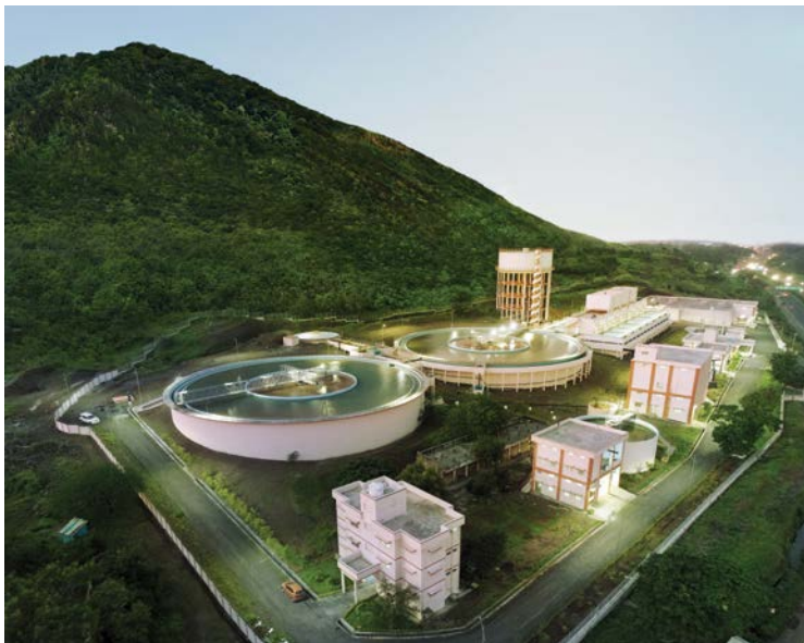
137 MLD Water Treatment Plant, Nashik, Maharashtra
