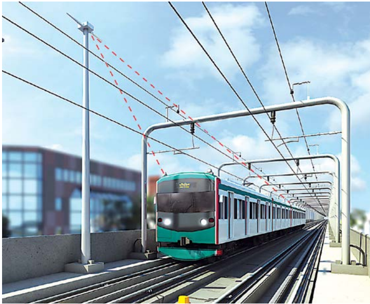
E&AM System Works, Dhaka Metro
