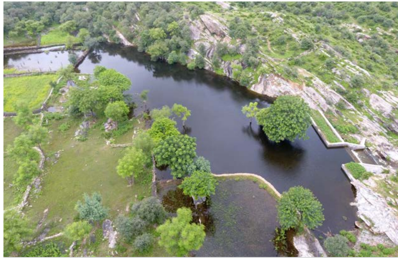
Anicut in Rajasthan - to help ease water stress in the area.
