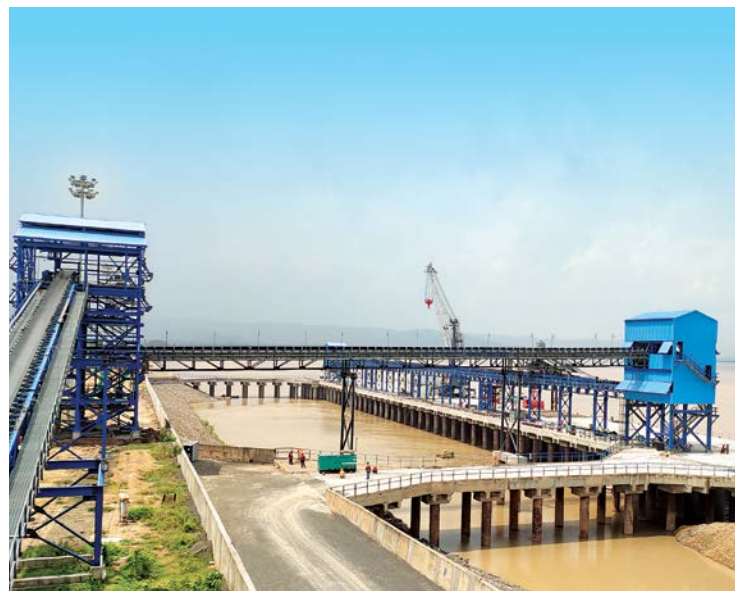
Multi-modal terminal at Sahibganj, Jharkhand
