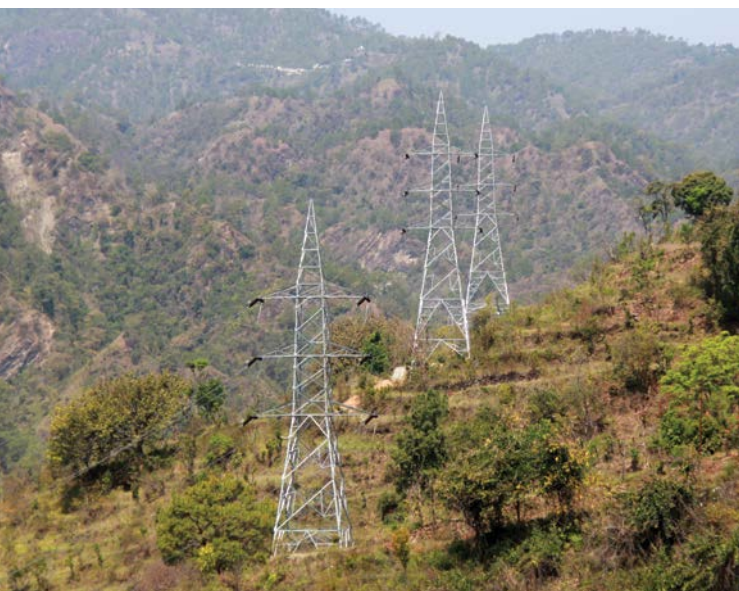
220 kV Transmission Line, Uttarakhand
