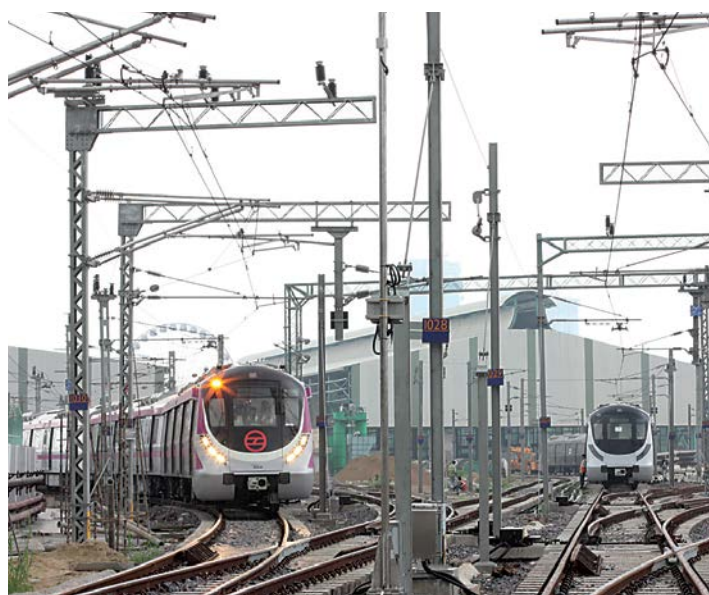
Overhead Electrification for Delhi Metro Phase 3
