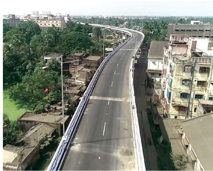
Bata Nagar Flyover, Kolkata, West Bengal
