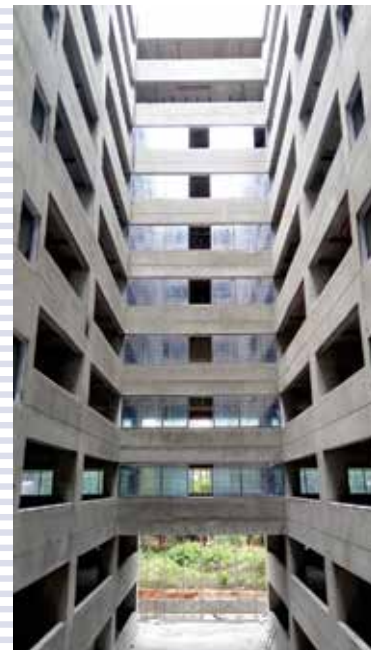
View of passage between 3A & 3B from the lobby
