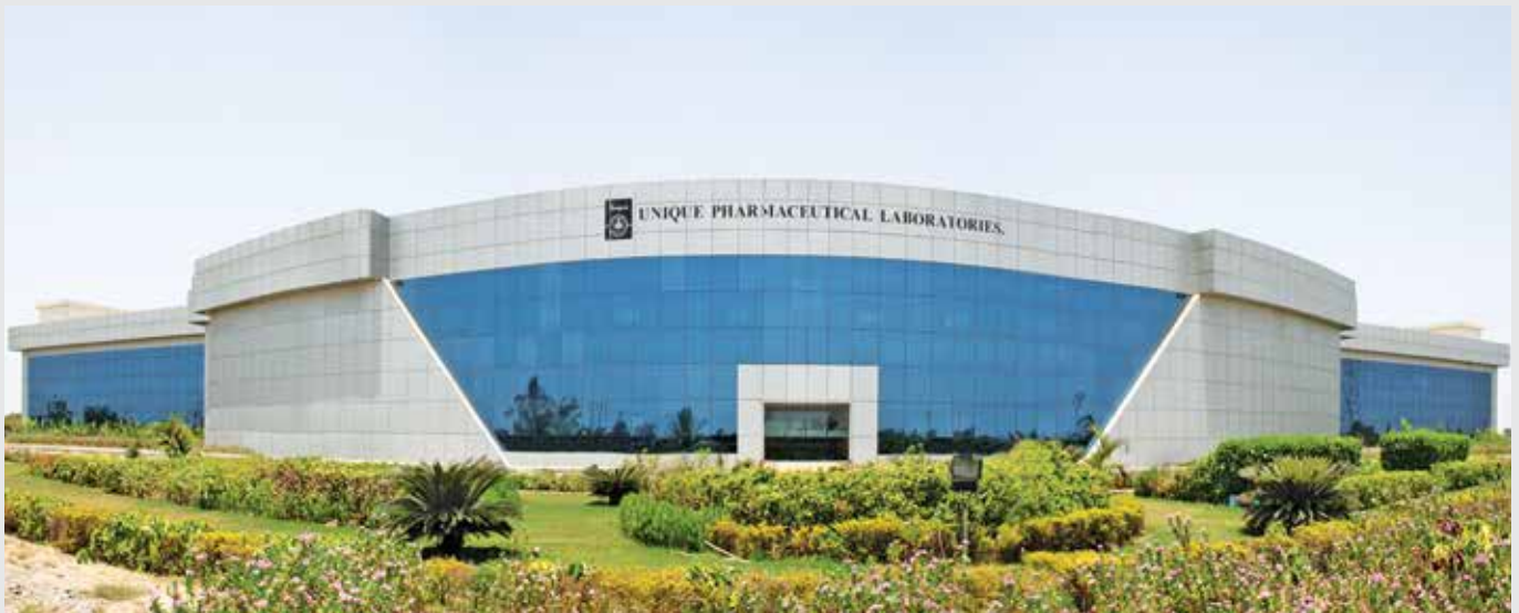
State-of-the-art Formulations manufacturing facility at Panoli, Gujarat
