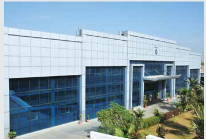
State-of-the-art Tablets and Lozenges manufacturing facility at Kadaiya, Daman
