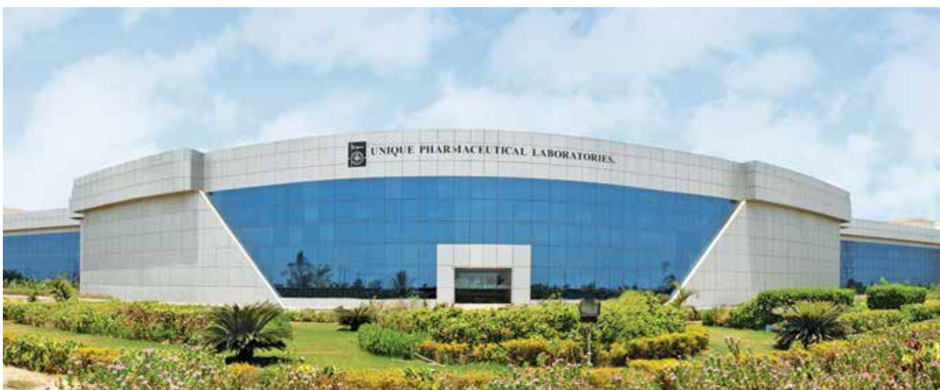
State-of-the-art Formulations manufacturing facility at Panoli, Gujarat
