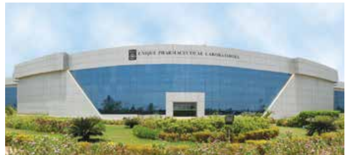
State-of-the-art Formulations manufacturing facility at Panoli, Gujarat
