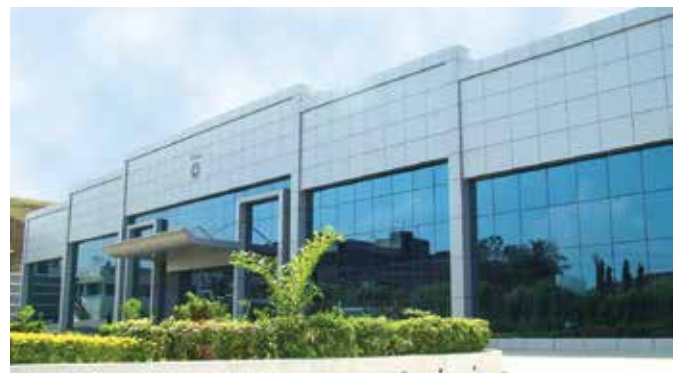
State-of-the-art Tablets and Lozenges manufacturing facility at Kadaiya, Daman
