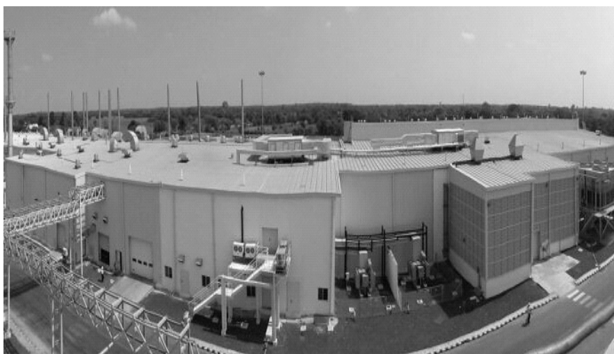
Factory Building for McCain Food India Pvt Ltd, Baliasan, Mehsana Dist. Gujarat
