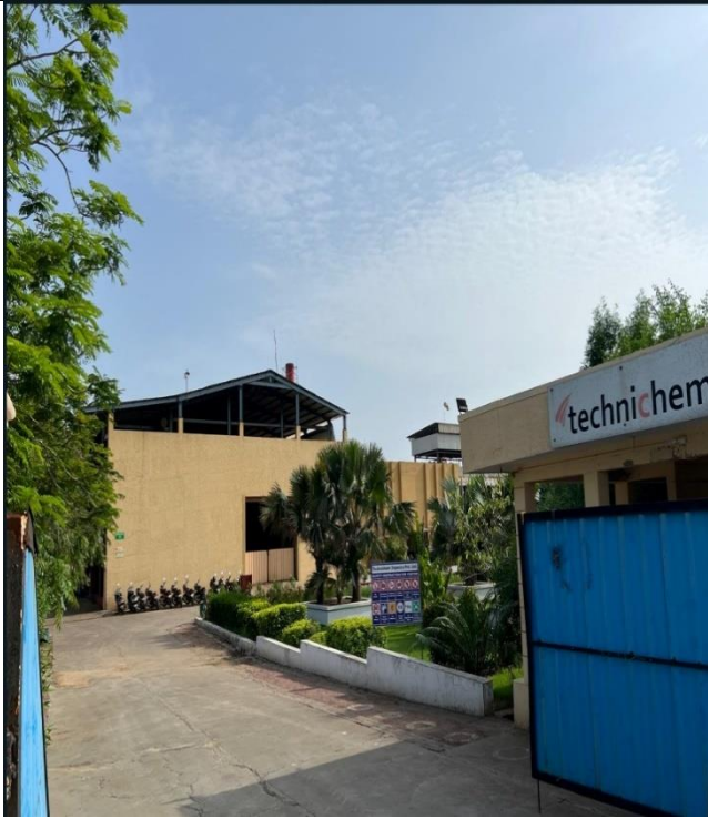
Entrance to Premises
