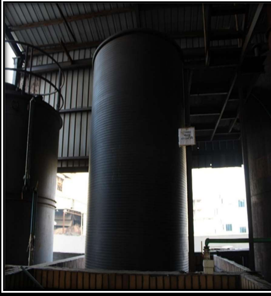
Machinery Name: Settling Tank Location In Plant: ETP Capacity: 50000LTR Use: In Etp for Effluent Storage After Treatment
