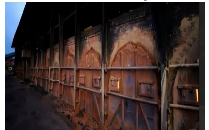
Battery with 32 Ovens
