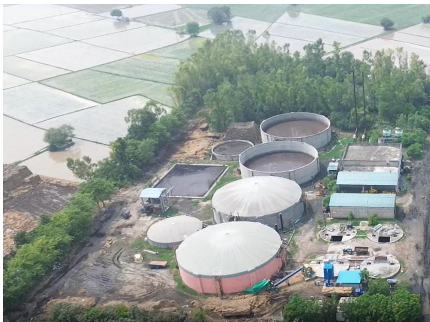
Bio-Gas Generation Plant
