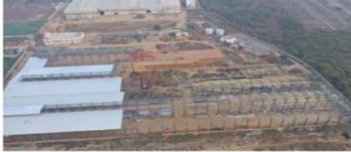
Phase II (Under Construction)
