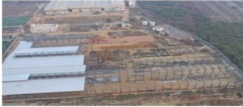
Phase II (Under Construction)
