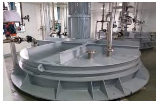
Blenders for the production of petroleum jellies at our Taloja Plant
