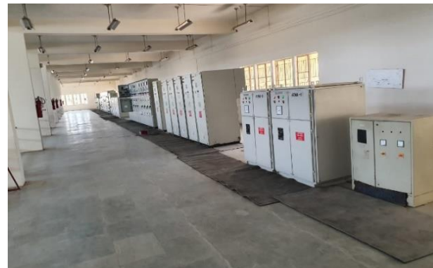
Gujrat Water Infrastructure Project (GWIL), Anjar, Kutch, Package-3
