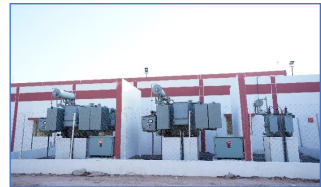
Gujrat Water Infrastructure Project (GWIL), Anjar, Kutch, Package-4
