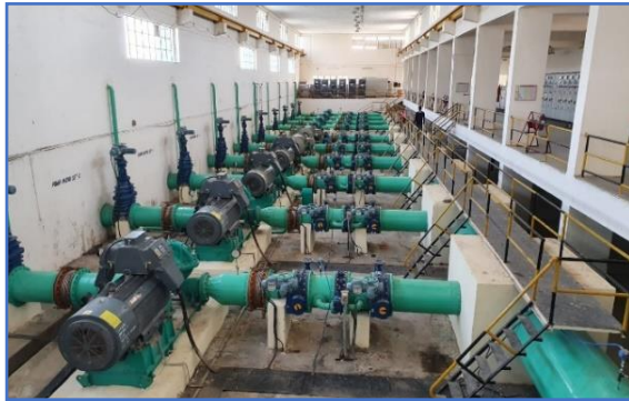
Gujrat Water Infrastructure Project (GWIL), Anjar, Kutch, Package-3
