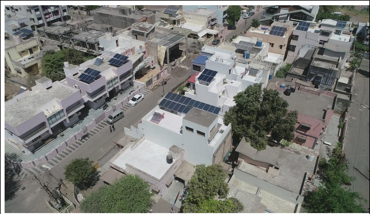
Residential Rooftop Projects
