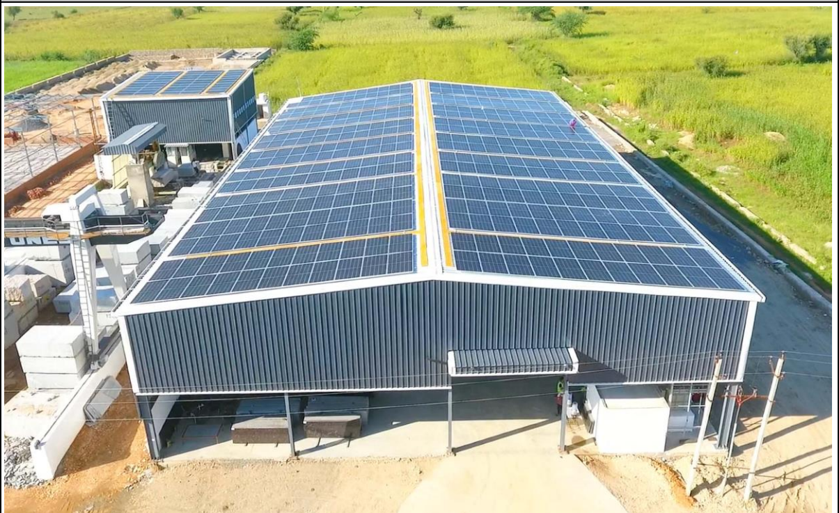
Commercial & Industrial Projects
