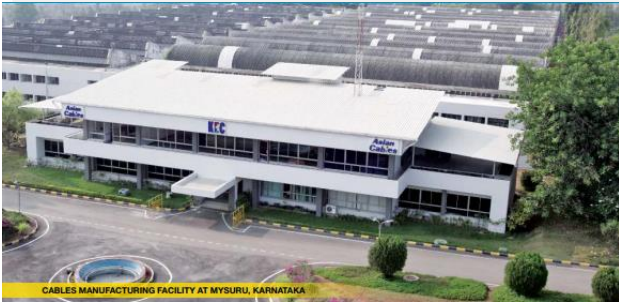
CABLES MANUFACTURING FACILITY AT MYSURU, KARNATAKA
