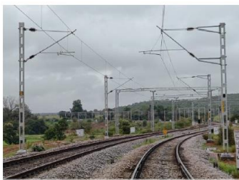
Hubli - Tinaighat Railway Electrification project, Karnataka
