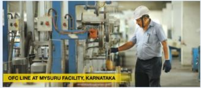
OFC LINE AT MYSURU FACILITY, KARNATAKA
