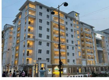
Construction of luxury residential project in Goa
