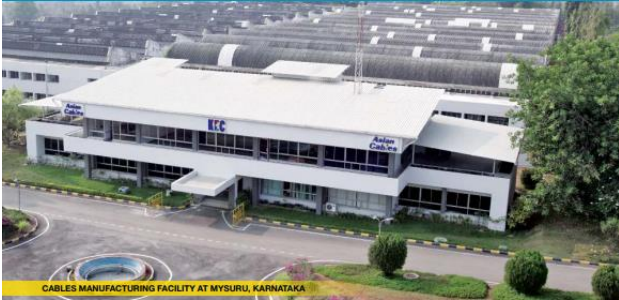
CABLES MANUFACTURING FACILITY AT MYSURU, KARNATAKA
