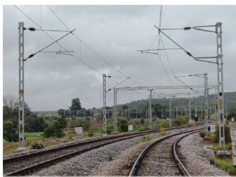
Hubli - Tinaighat Railway Electrification project, Karnataka
