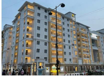
Construction of luxury residential project in Goa
