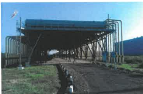
CS - 8 Gas After Cooler
