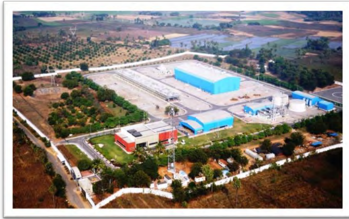
Aerial view of compressor station – CS 3
