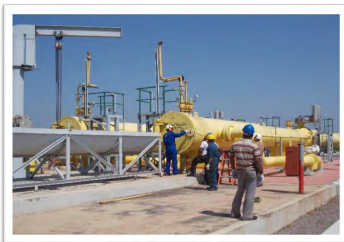
Pig Launcher and Receiver – CS5
