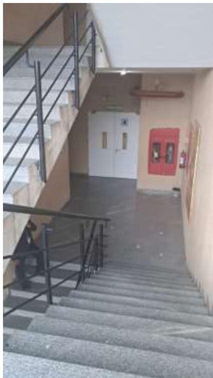
Internal View of stairwell in Subject Tower
