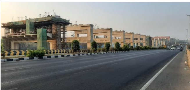
Images of construction progress
