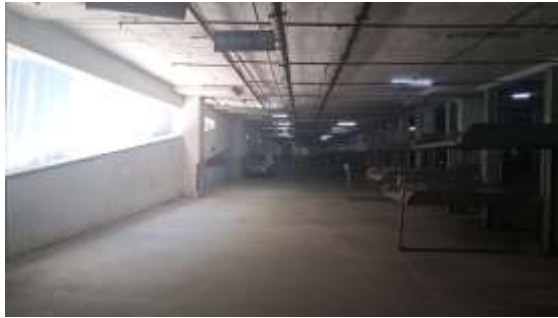
View of basement and stack parking in Subject Tower
