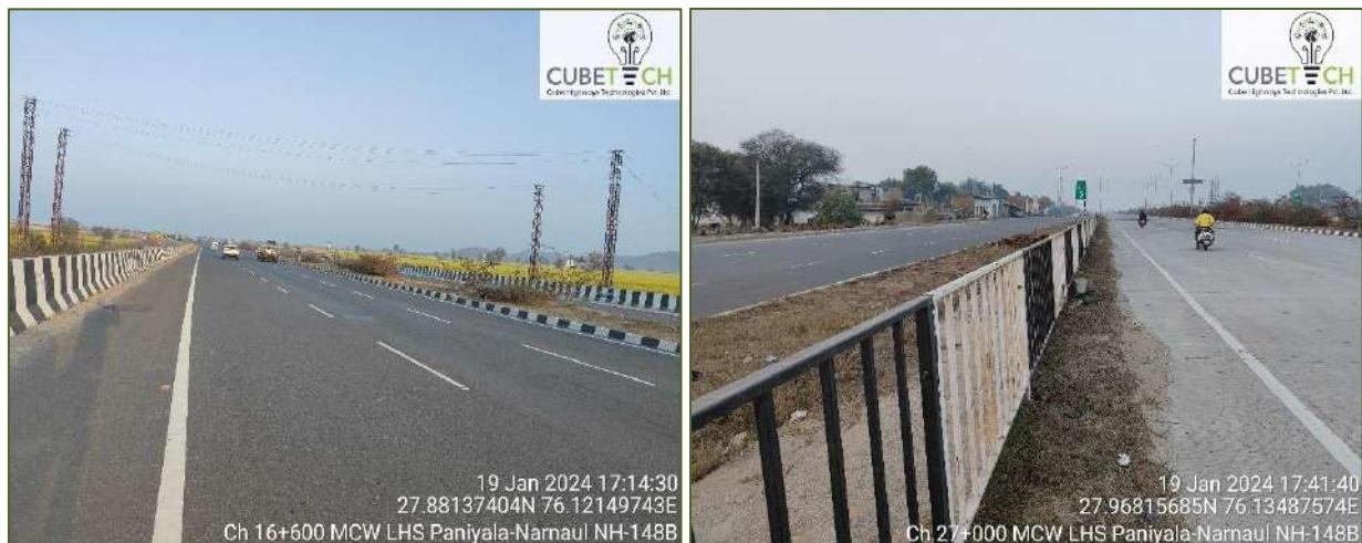
Figure 3-4: Safety crash barrier (MBCB) along the project stretch
