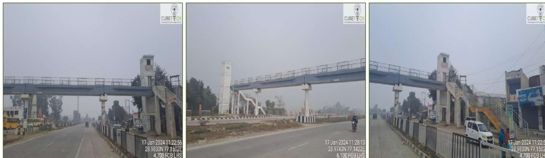
Figure 4-4: Foot Over Bridge at km 4.700 and km 5.980
