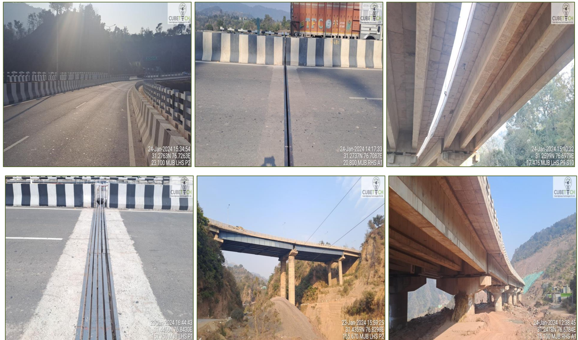
Figure 4-1: Condition of Major Bridge
