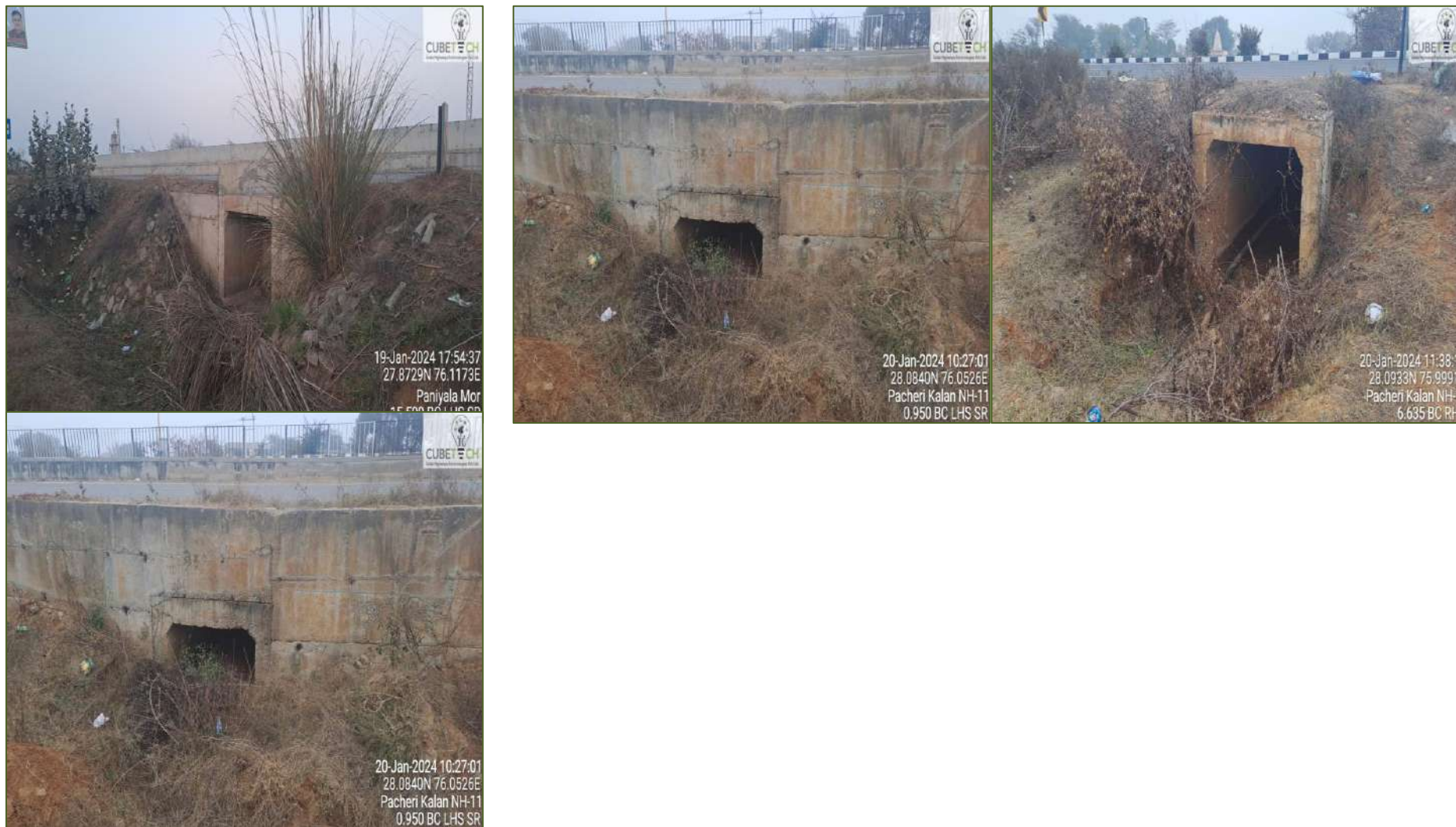
Figure 4-5: Condition of Culvert
