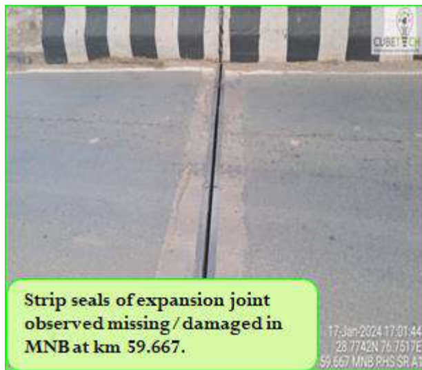
Figure 4-1: Condition of Minor Bridges
