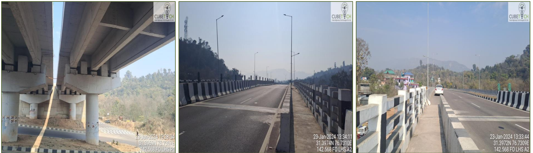
Figure 4-4: Condition of Flyover
