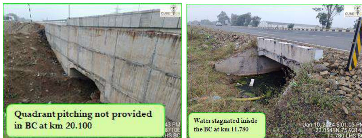
Figure 4-8: Condition of Culverts
