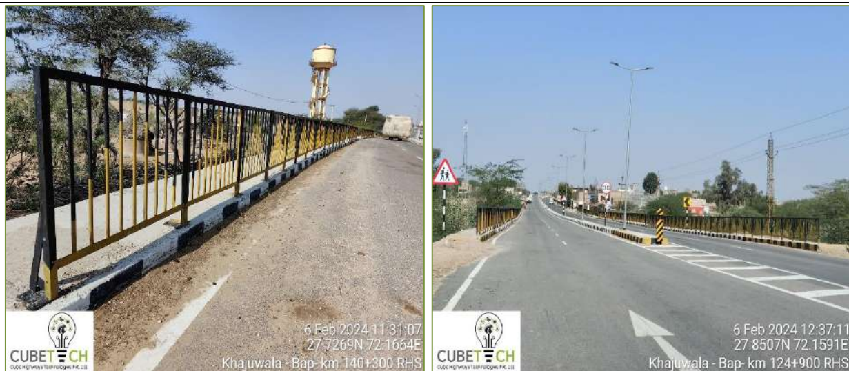
Figure 3-7: Pedestrian guard rail
