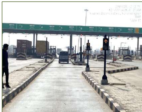
Figure 3-14: Over Head Lane Signal (OHLS).
