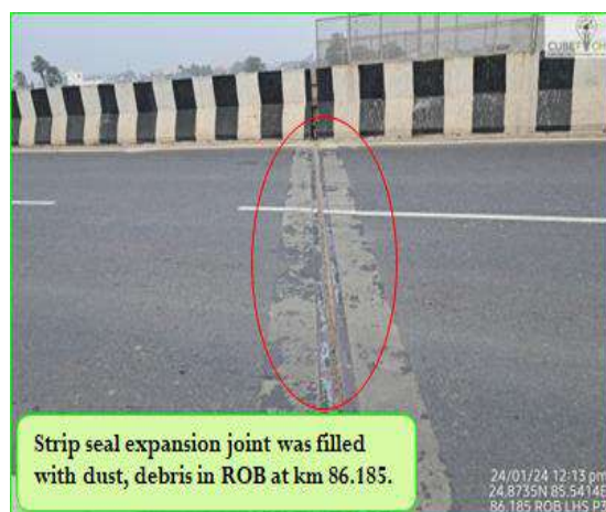
Figure 4-2: Condition of Road Over Bridges
