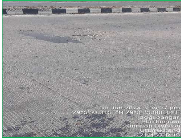
Figure: Scaling
