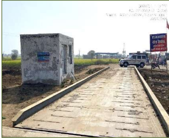
Figure 3-16: Static Weigh Bridge (SWB).
