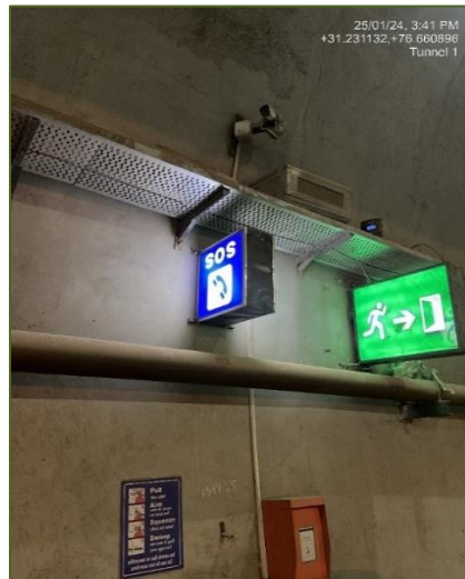
Figure 3-42: Tunnel-1 ECB.
