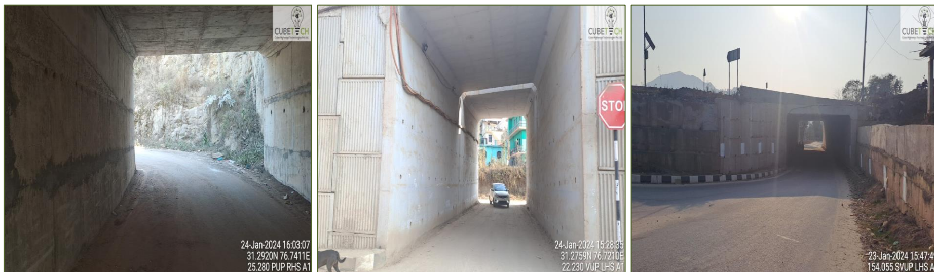
Figure 4-6: Condition of Underpasses
