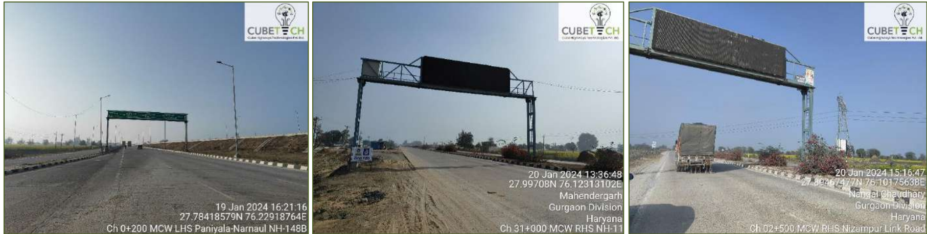
Figure 3-5: Overhead & Cantilever Gantry boards
