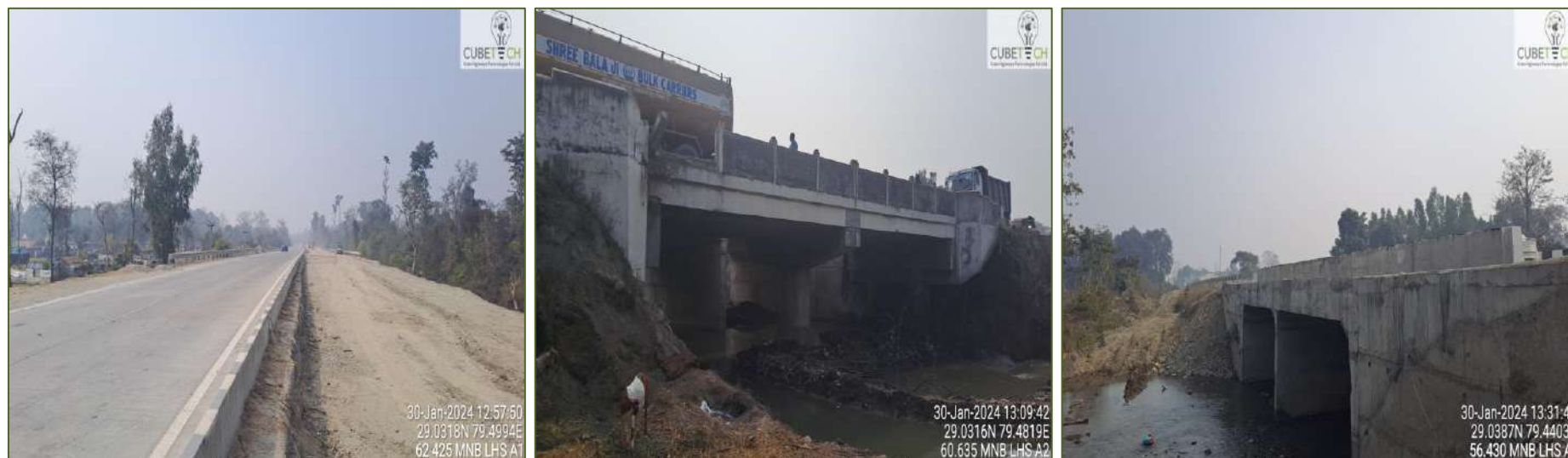
Figure 4-2: Condition of Minor Bridges
