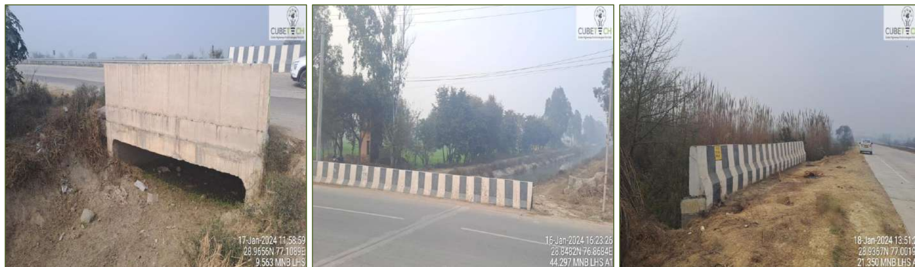
Figure 4-1: Condition of Minor Bridges
