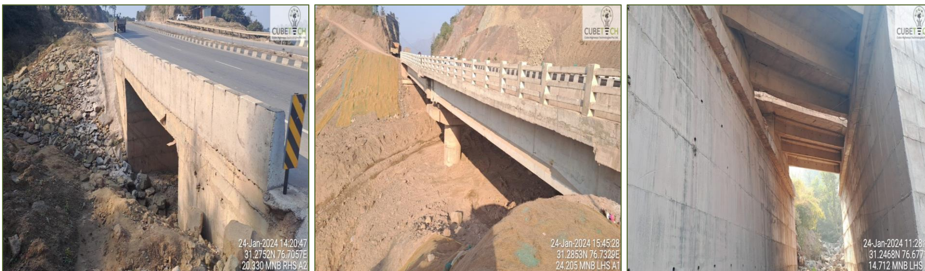
Figure 4-2: Condition of Minor Bridge
