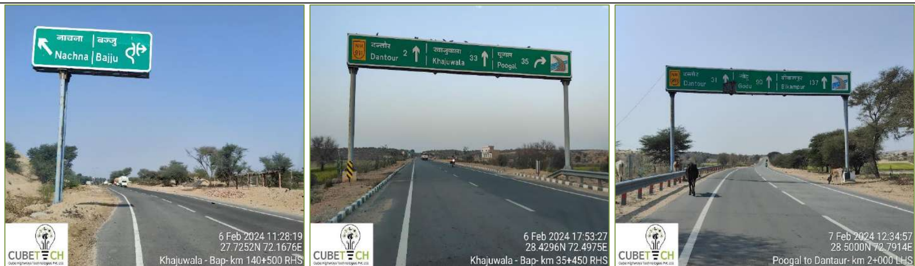
Figure 3-6: Overhead & Cantilever Gantry boards
