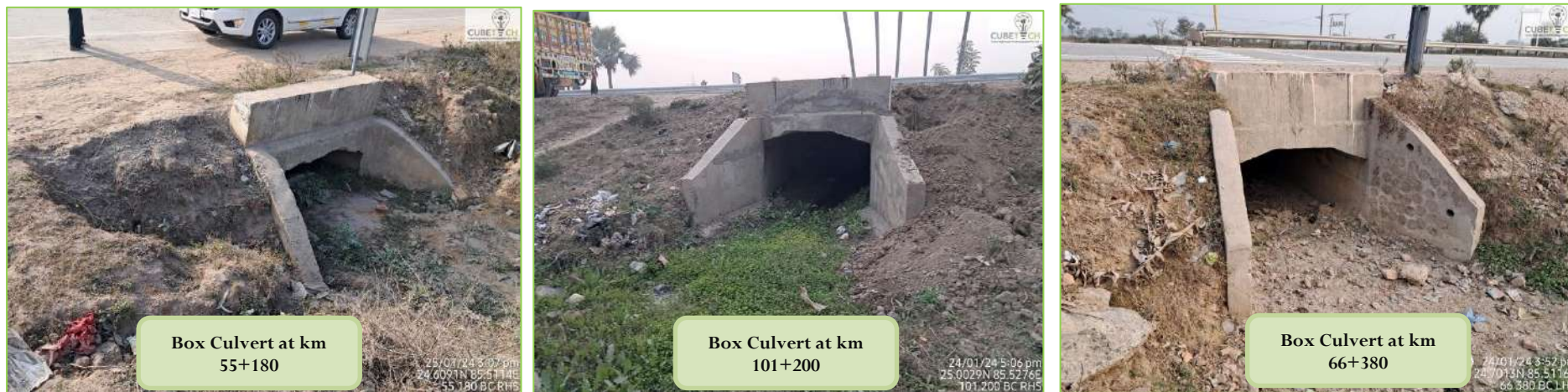
Figure 4-7: Condition of Box Culverts
