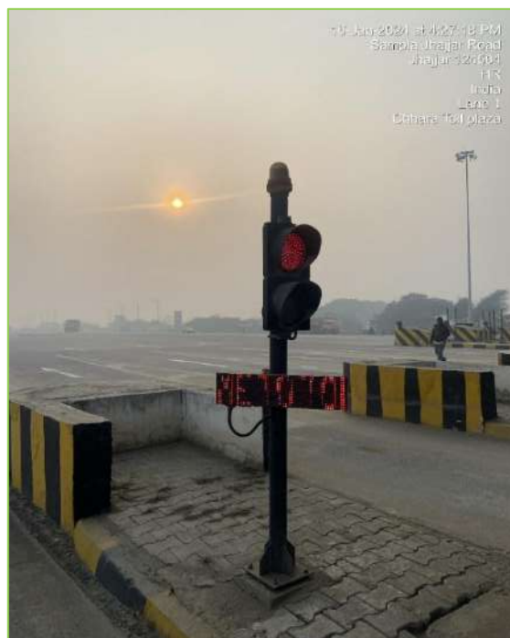
Figure 3-14: Traffic Light (TL) and User Fare Display (UFD).
