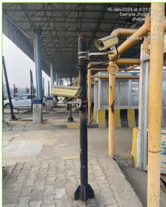
Figure 3-15: LPIC and ICS Cameras.
