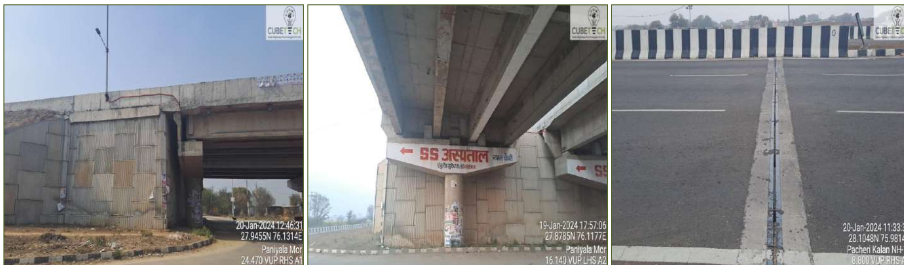
Figure 4-3: Condition of Vehicular Underpasses
