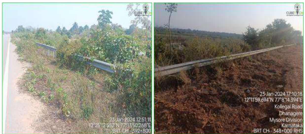
Figure 3-5: Safety crash barrier (MBCB) along the project stretch
