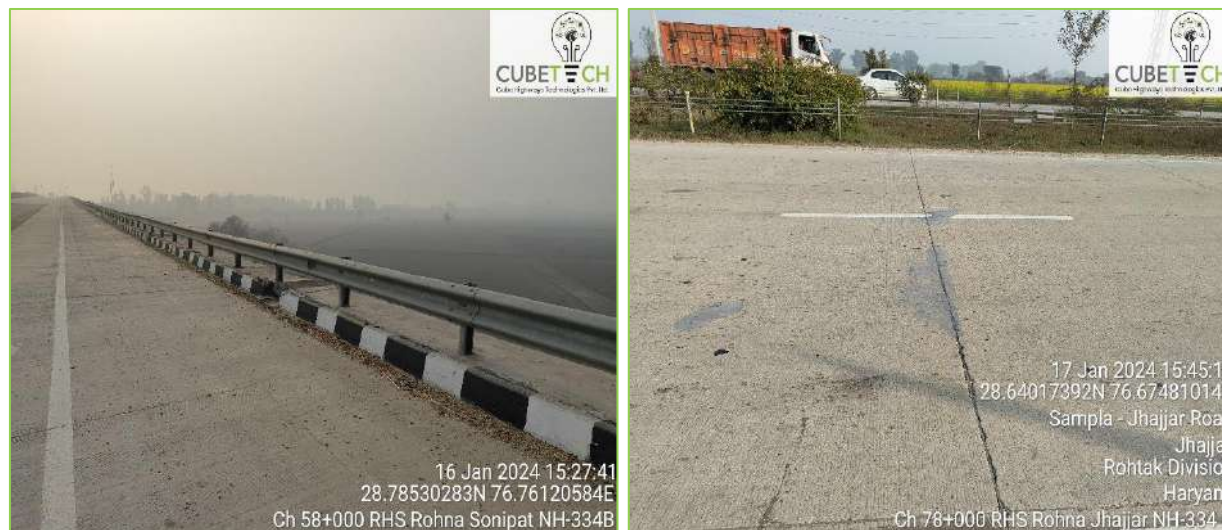
Figure 3-4: Crash barrier along the project stretch
