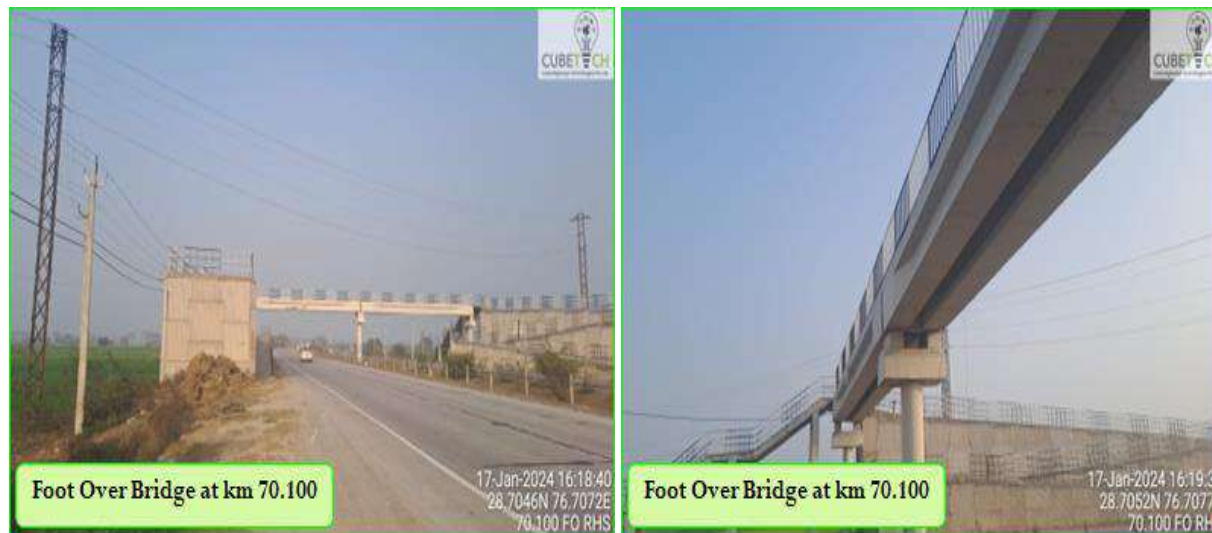
Figure 4-4: Condition of Foot Over Bridge
