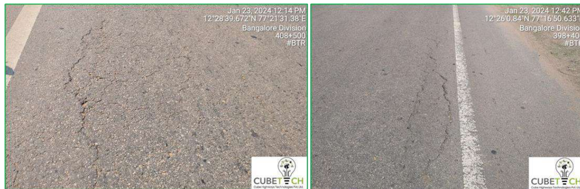
Figure 7-7: Alligator Cracks
