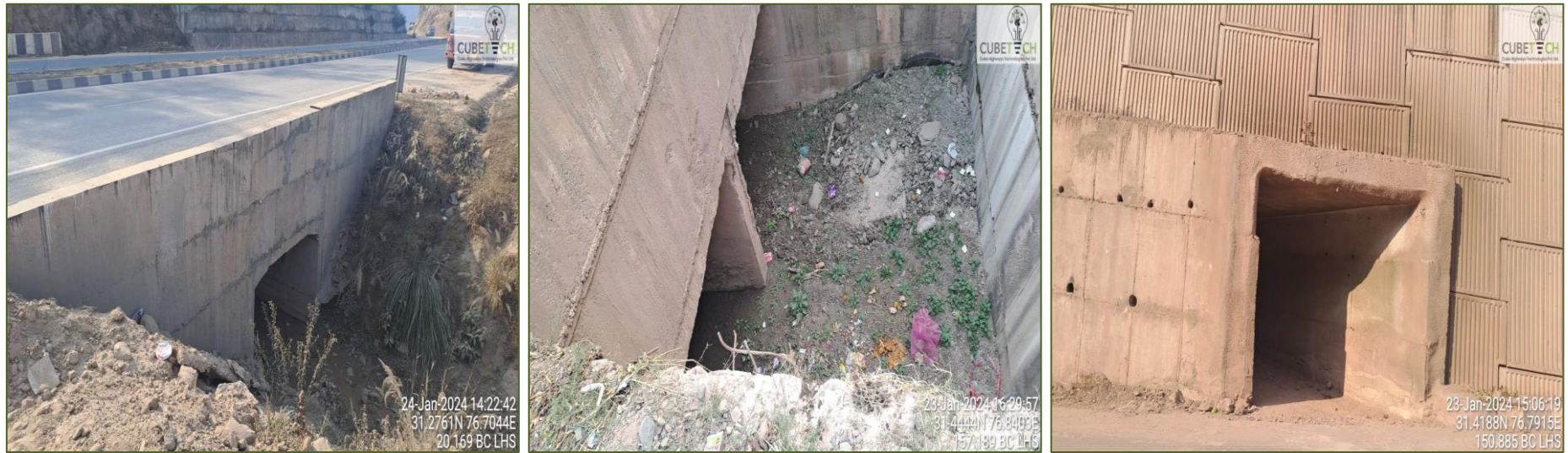
Figure 4-7: Condition of Culverts
