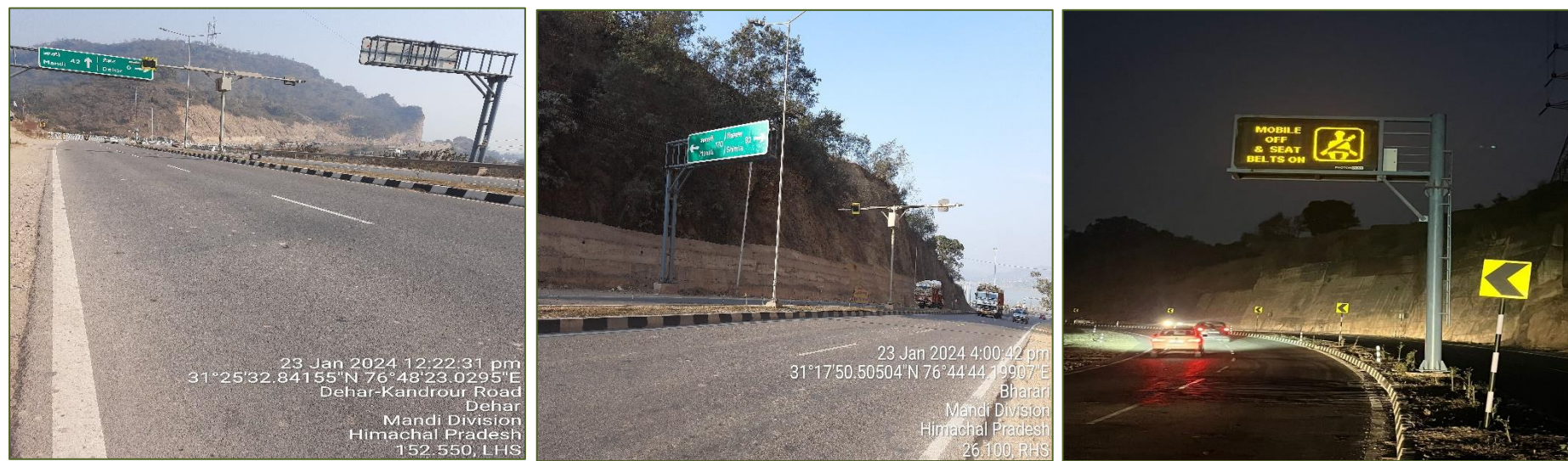
Figure 3-5: Overhead & Cantilever Gantry boards and VMS
