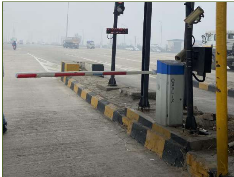
Figure 3-12: Boom Barrier.
