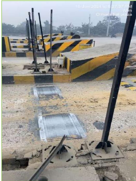
Figure 3-18: Medium Speed Weigh in Motion (MSWIM).
