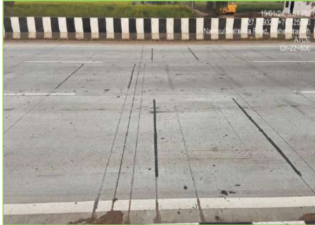
Figure 3-22: PLP Based ATCC.
