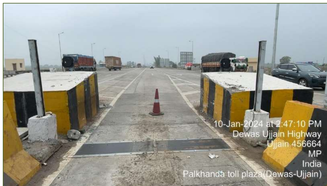
Figure 3-22: Medium Speed Weigh in Motion (MSWIM)
