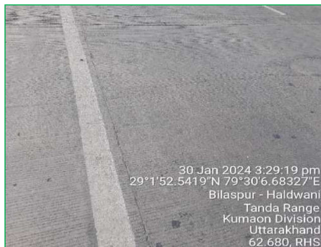
Figure 0-2: Transverse Cracks
