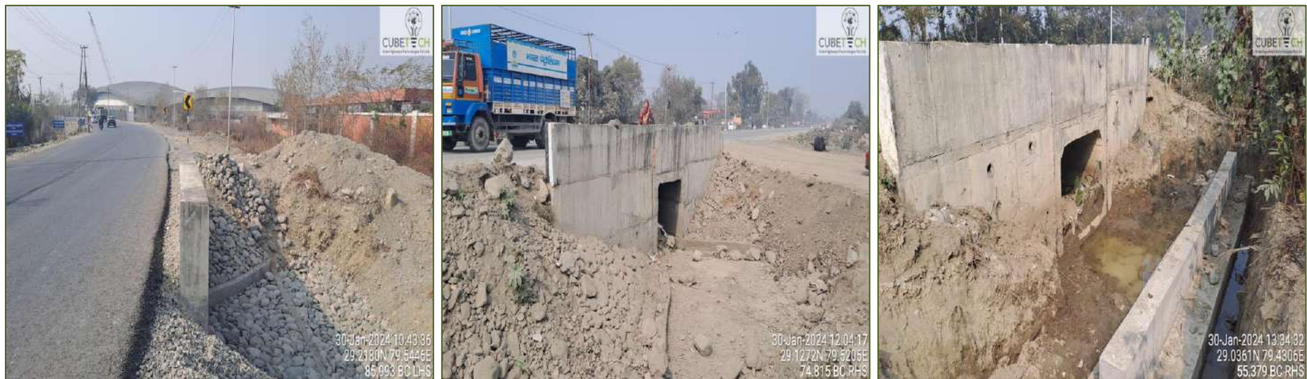
Figure 4-6: Condition of Culverts
