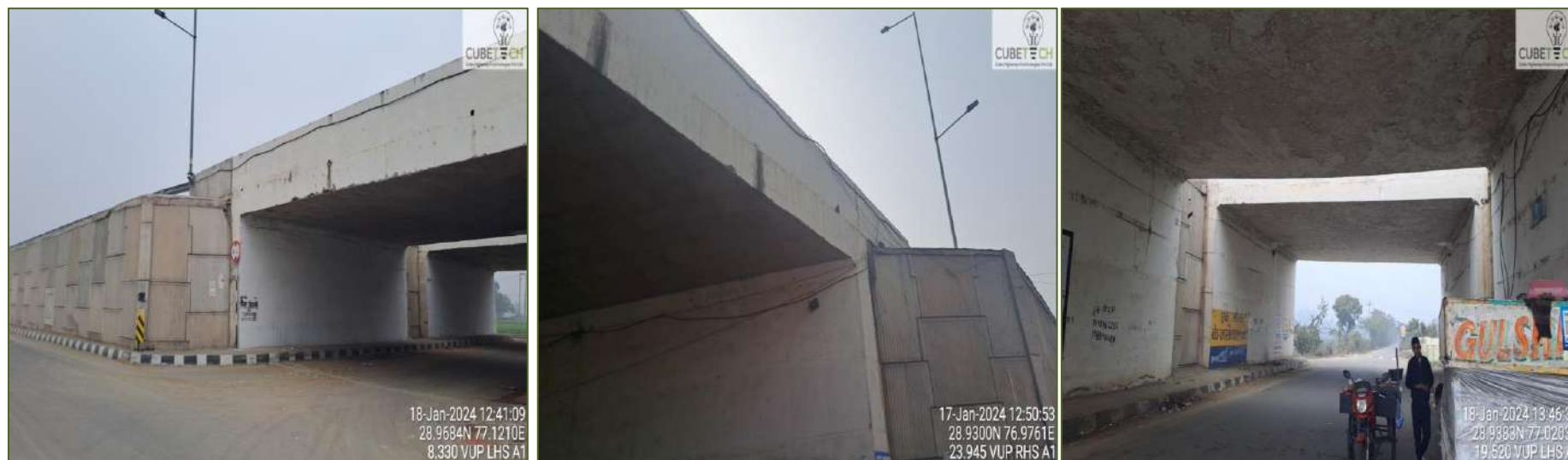
Figure 4-5: Condition of Vehicular Underpasses
