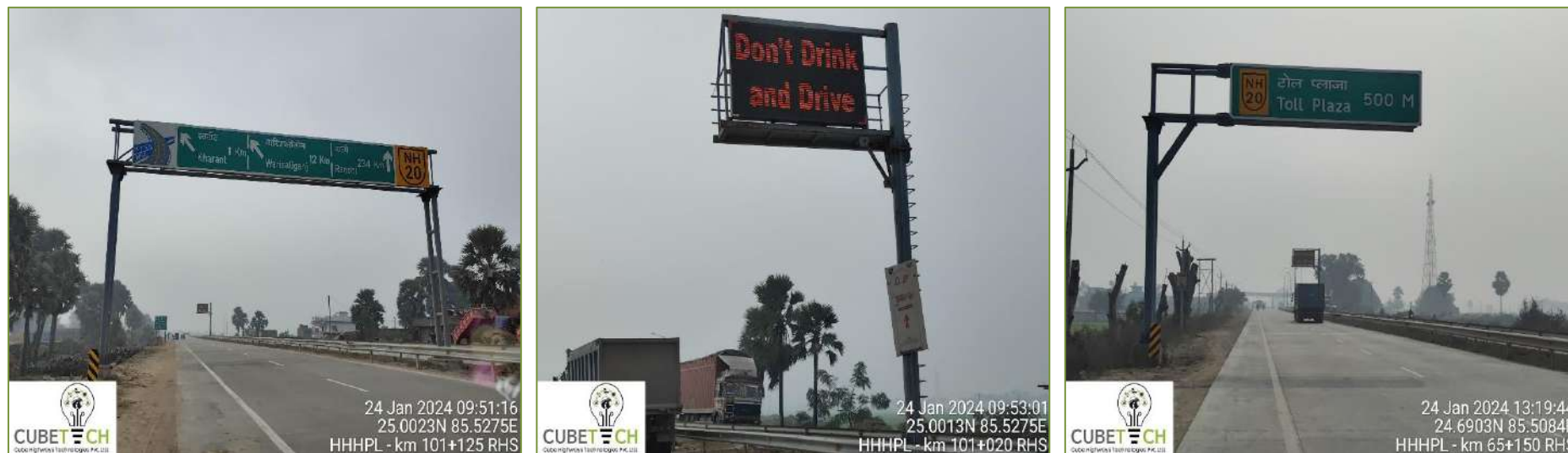
Figure 3-6: Overhead & Cantilever Gantry boards and VMS
