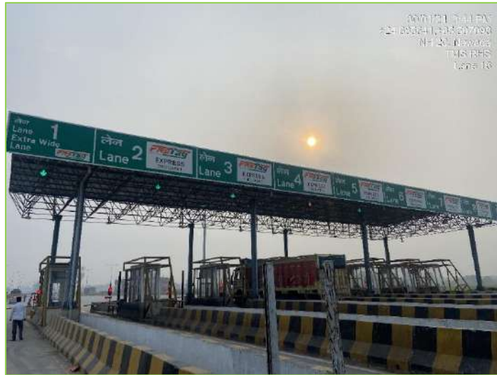
Figure 3-21: Over Head Lane Signal (OHLS).
