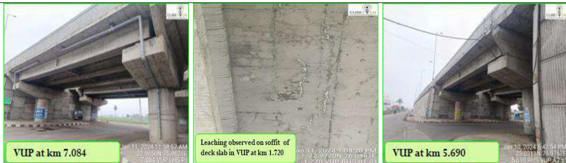
Figure 4-5: Condition of VUPs
