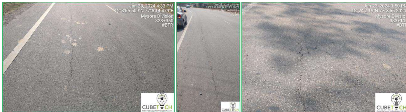
Figure 7-6: Longitudinal Cracks
