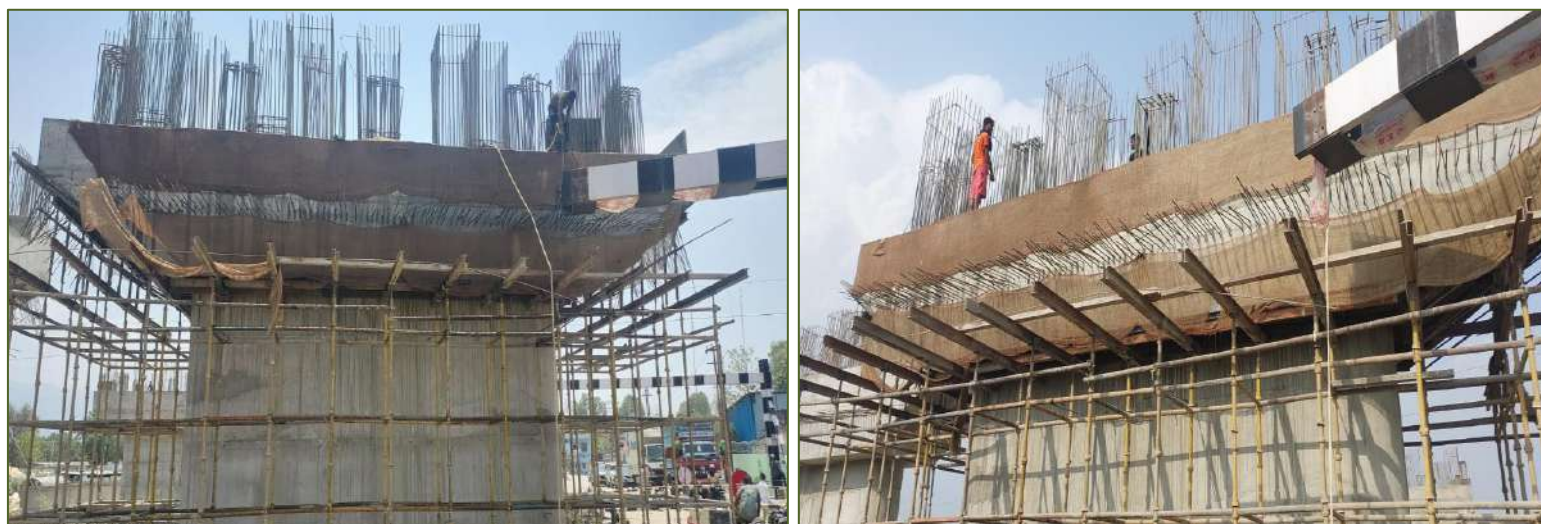
Figure 4-3: Progress of ROB
