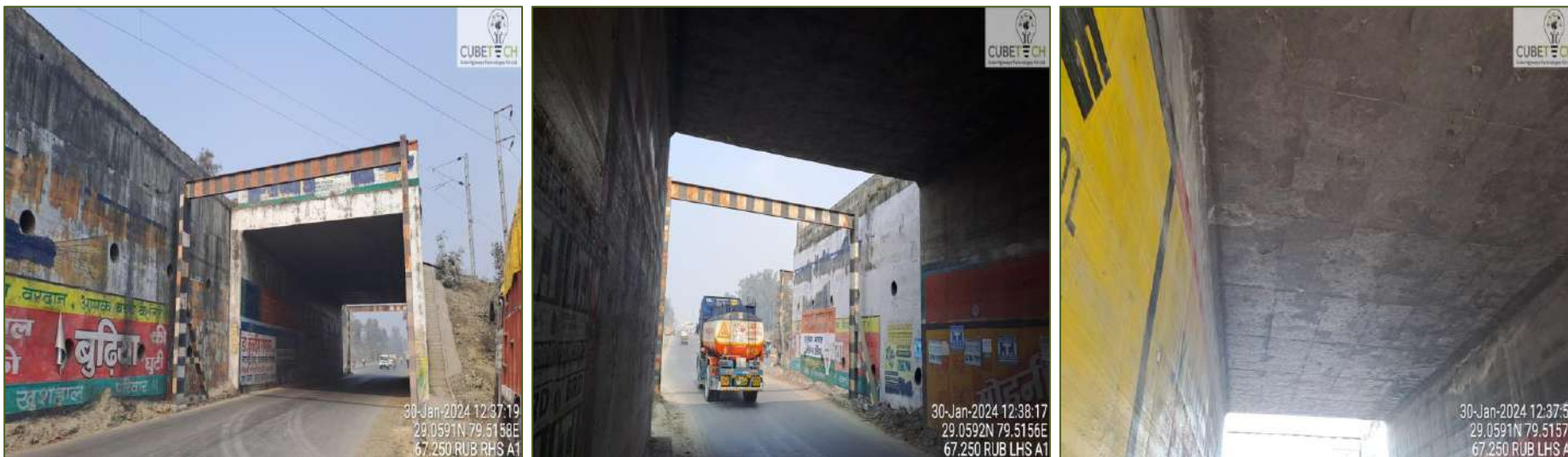
Figure 4-4: Condition of RUB
