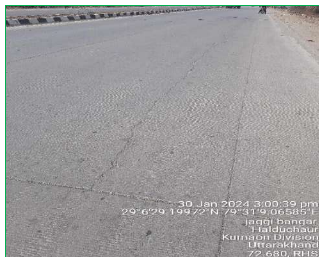
Figure 0-1: Longitudinal Cracks
