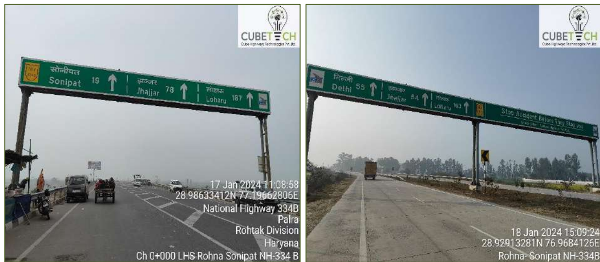
Figure 3-5: Overhead & Cantilever Gantry boards and VMS
