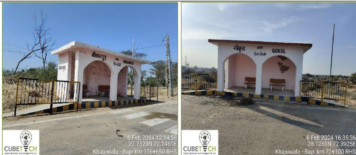
Figure 3-10: Bus bays / shelters
