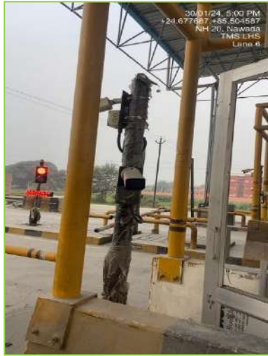
Figure 3-20: LPIC and ICS Cameras.
