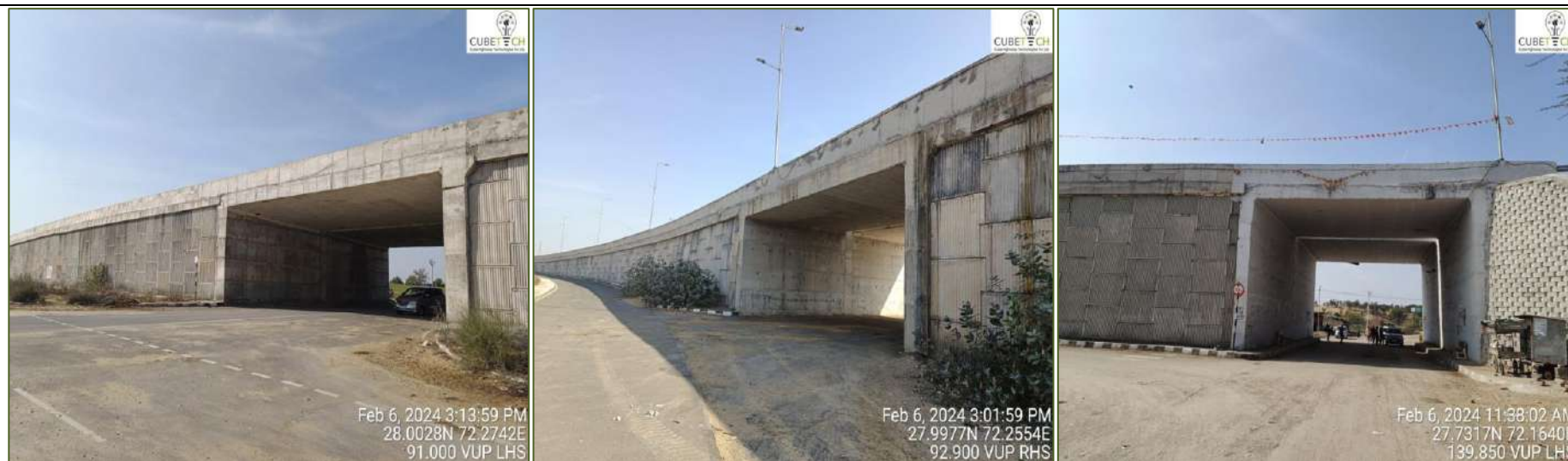
Figure 4-2: Condition of VUPs
