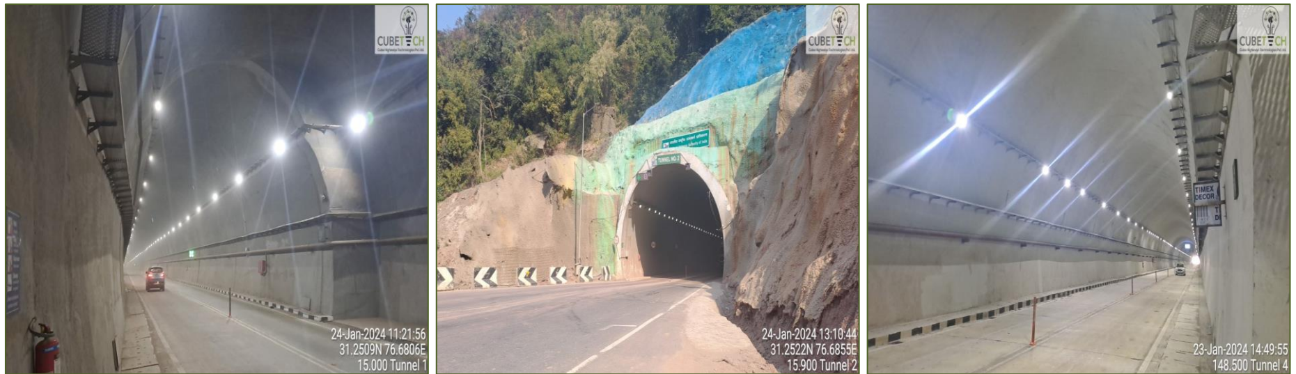
Figure 4-5: Condition of Tunnels
