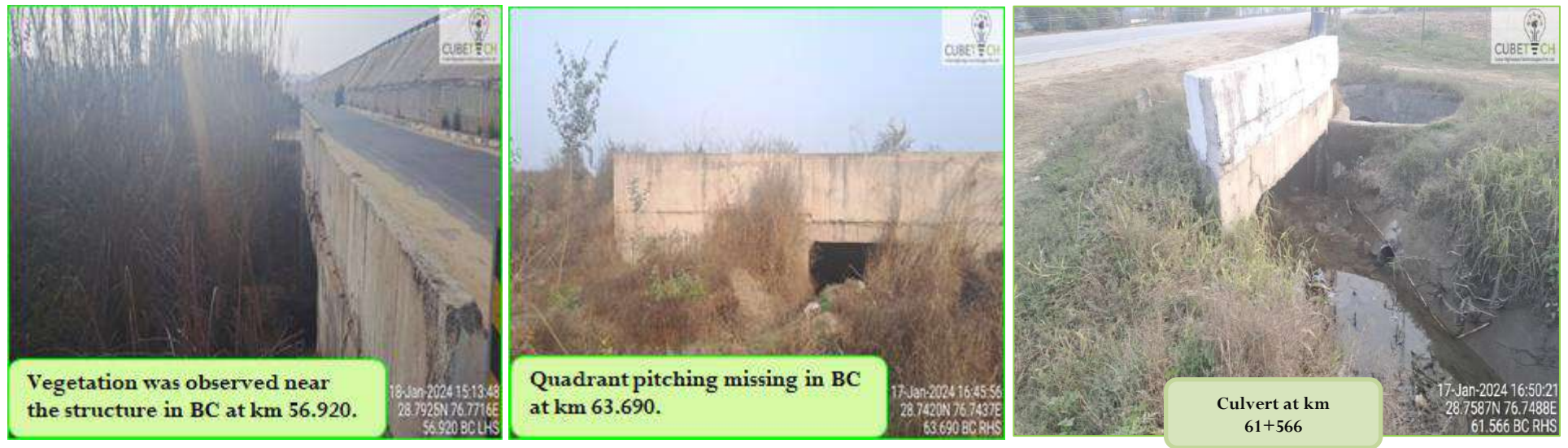
Figure 4-6: Condition of Culverts
