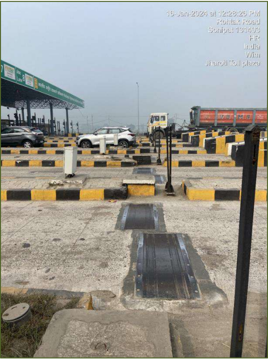
Figure 3-17: Medium Speed Weigh in Motion (MSWIM).
