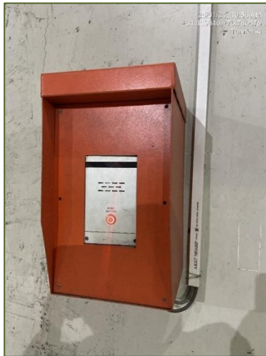
Figure 3-50: Tunnel-4 ECB.
