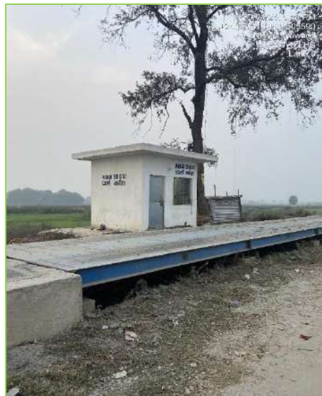
Figure 3-23: Medium Speed Weigh in Motion (MSWIM).
