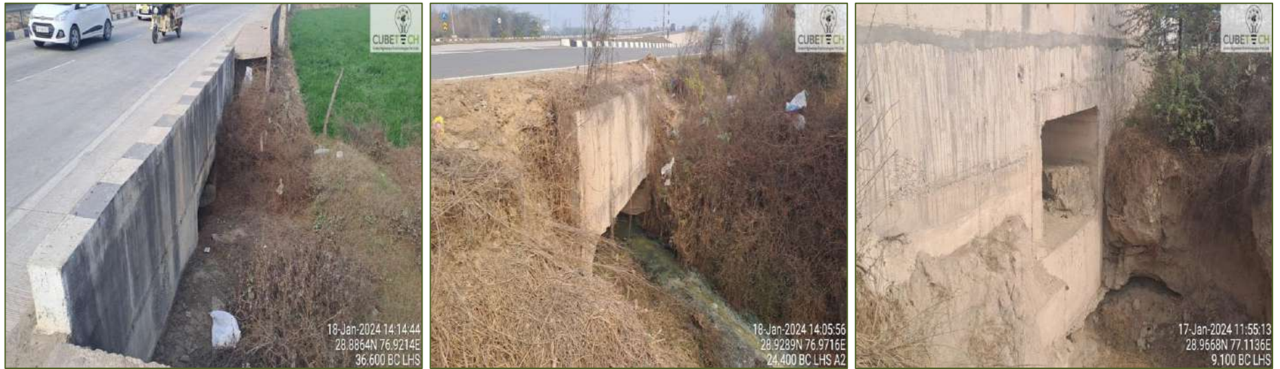
Figure 4-7: Condition of Culverts
