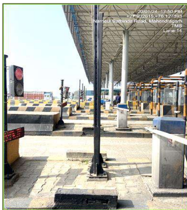
Figure 3-10: AVC Height Sensors
