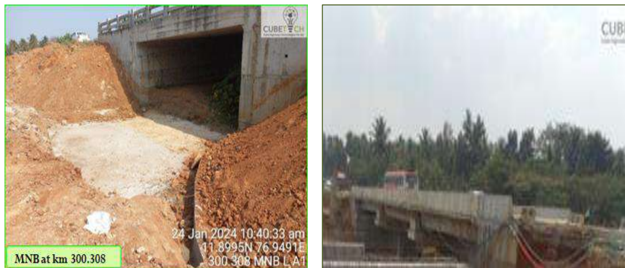
Figure 4-2: Condition of Minor Bridges at km 300+308 & 443+075
