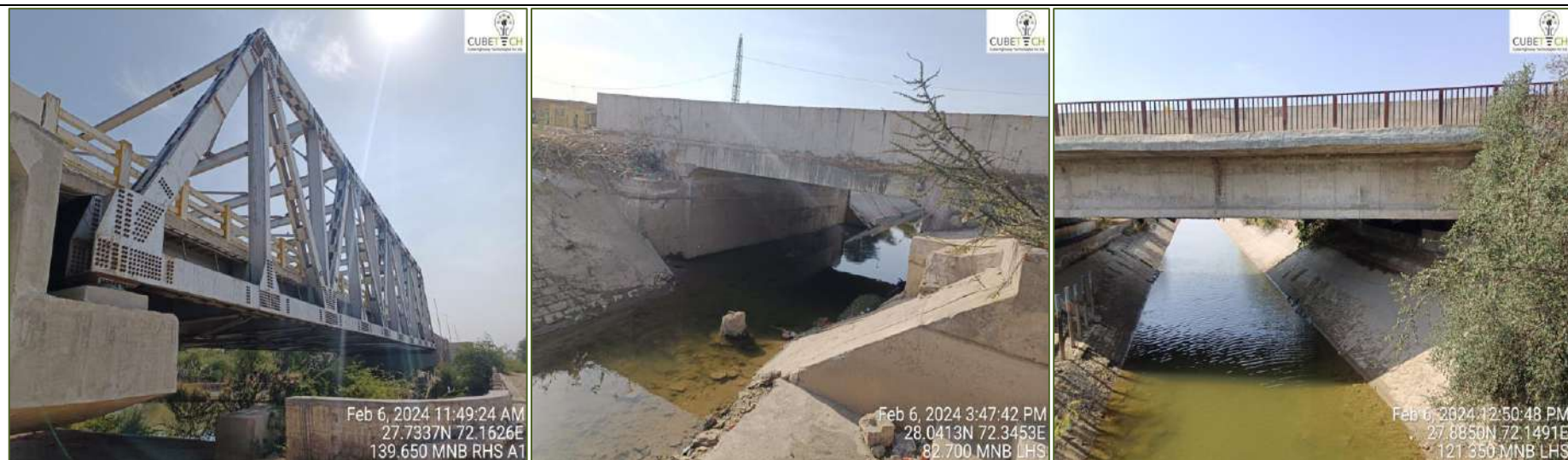
Figure 4-1: Condition of Minor Bridges
