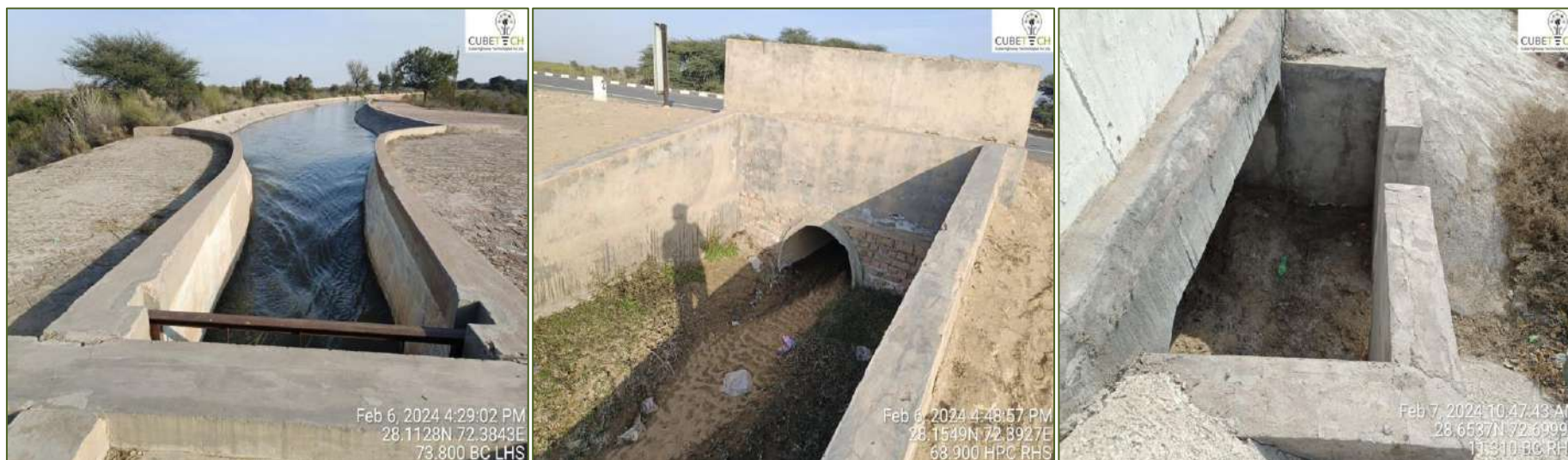
Figure 4-3: Condition of Box Culverts
