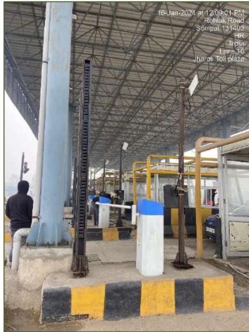
Figure 3-11: AVC IR Sensor.
