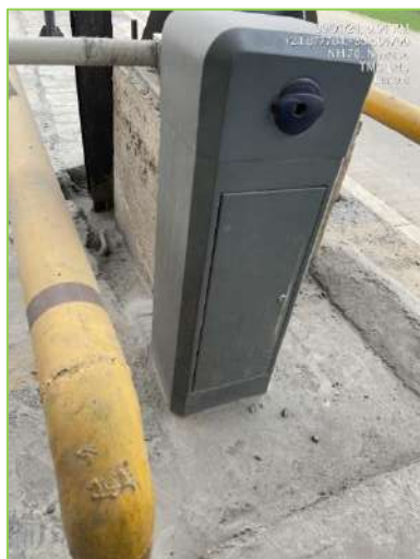
Figure 3-18: Boom Barrier.
