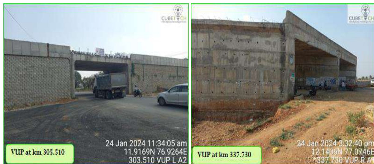
Figure 4-4: Condition of VUPs
