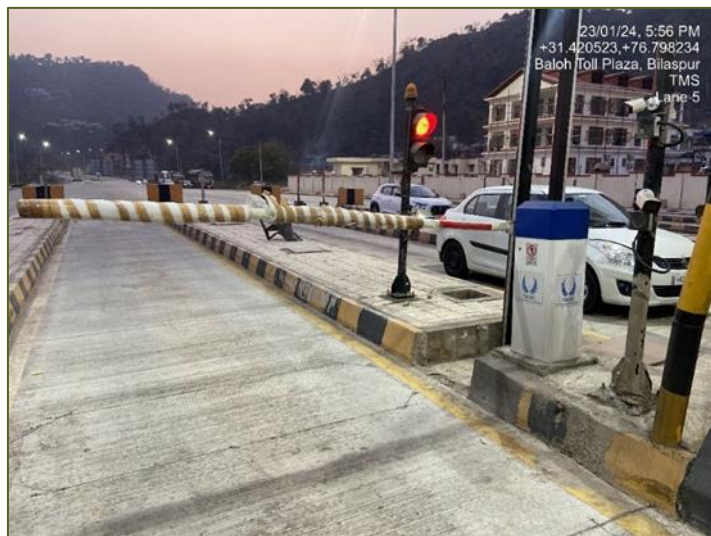
Figure 3-12: Boom Barrier.
