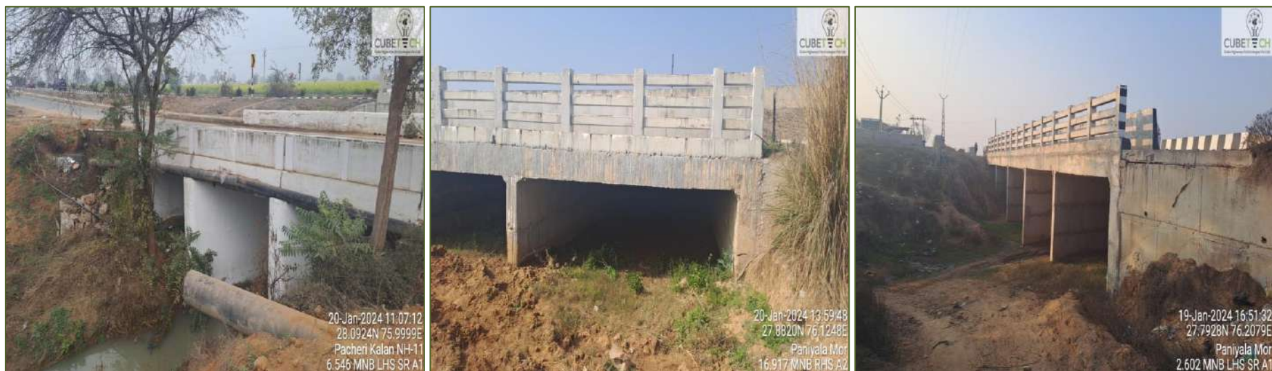
Figure 4-2: Condition of Minor Bridges
