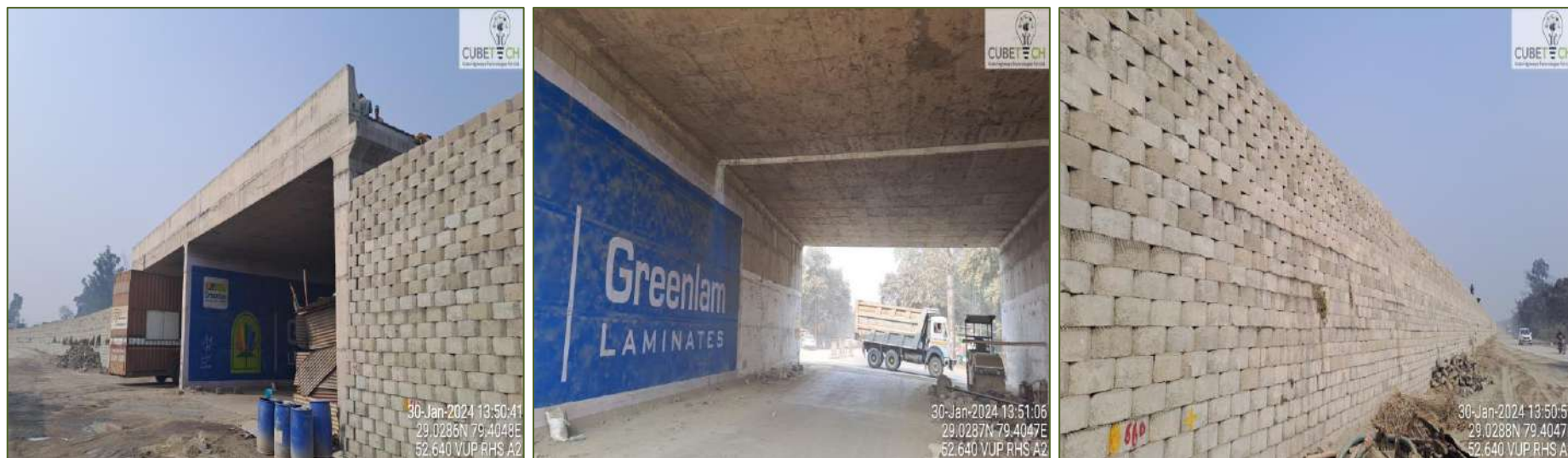
Figure 4-5: Condition of Vehicular Underpass
