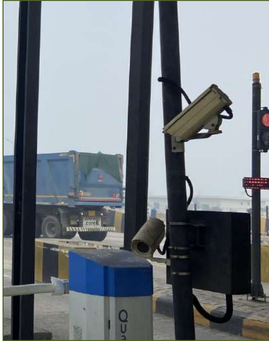
Figure 3-14: LPIC and ICS Cameras.
