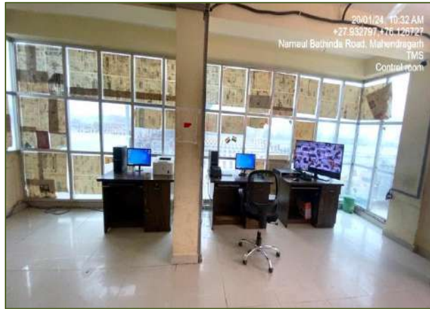
Figure 3-18: Workstations at Control room.
