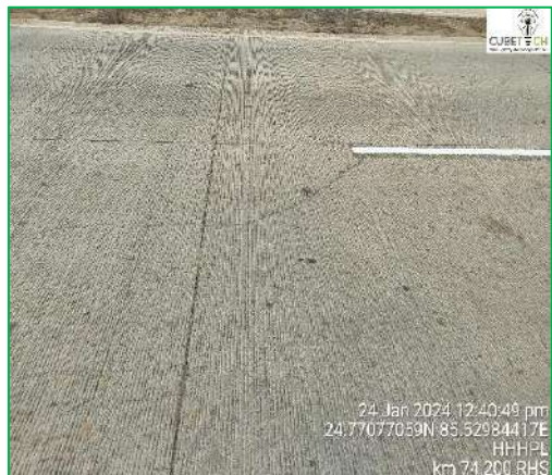
Figure: Corner Break
