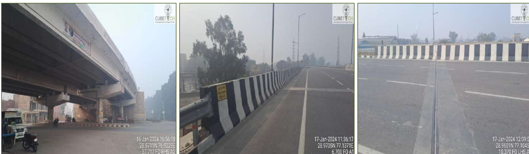
Figure 4-3: Condition of Flyover
