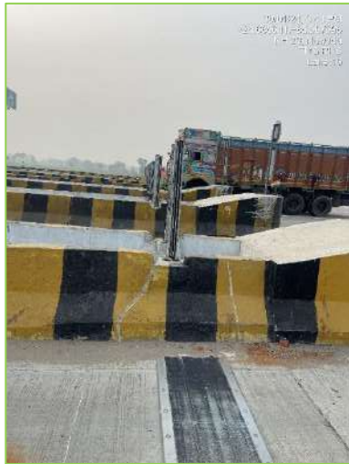
Figure 3-23: Medium Speed Weigh in Motion (MSWIM).
