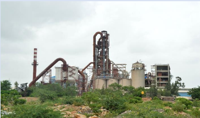
Capex 1 million Ton in Progress...
