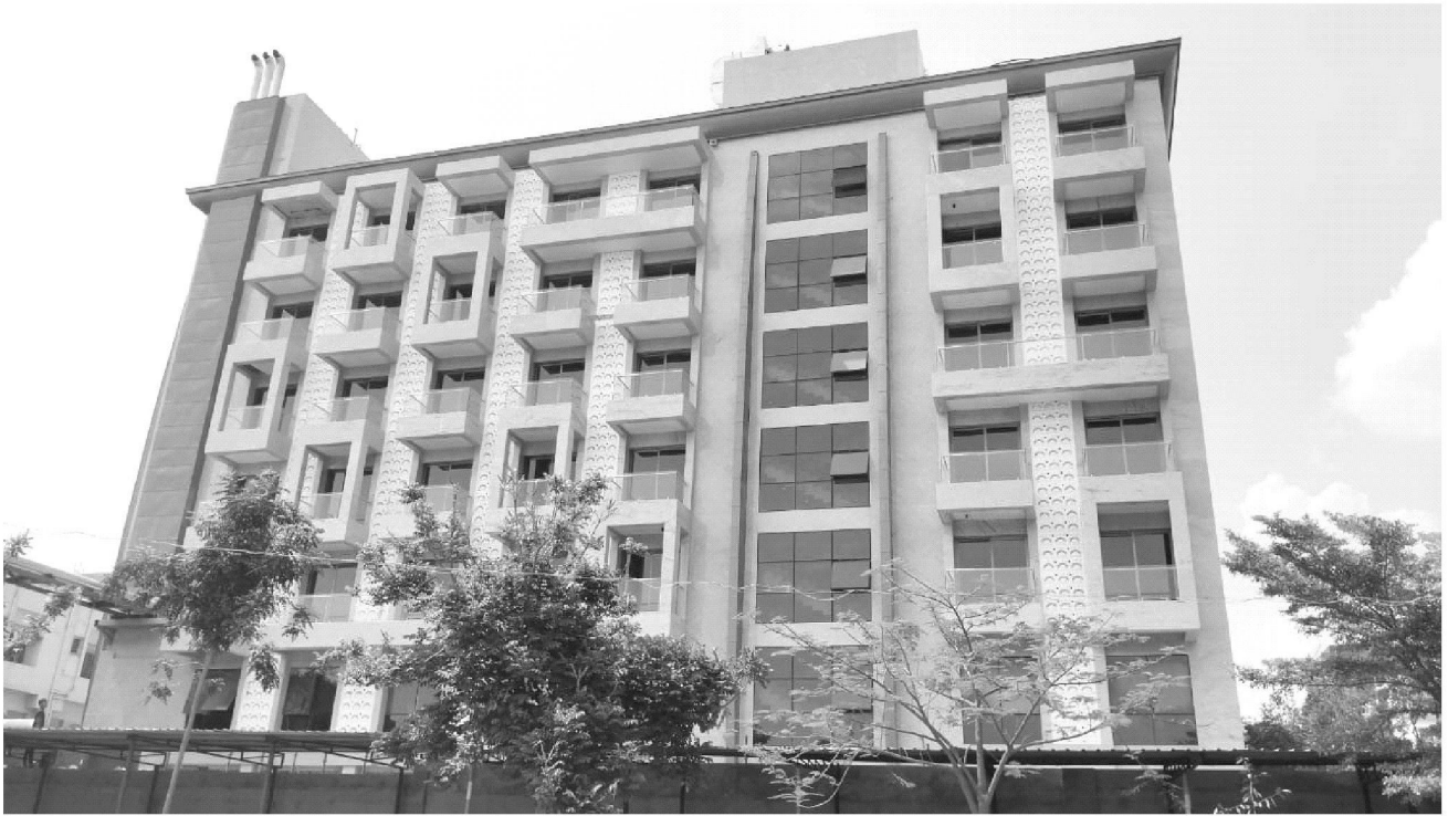
Institutional Building for M/s C.I.S.C.E -Council for the Indian School Certificate Examination (Regional Institute) at Habsiguda, Hyderabad
