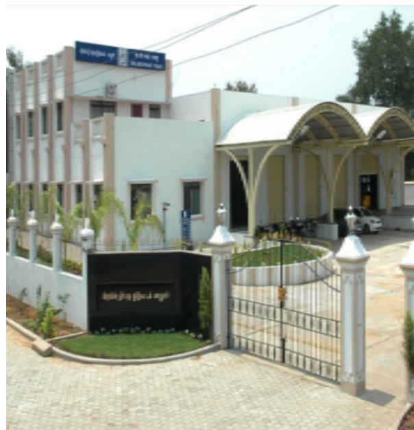
Railneer Plant Palur
