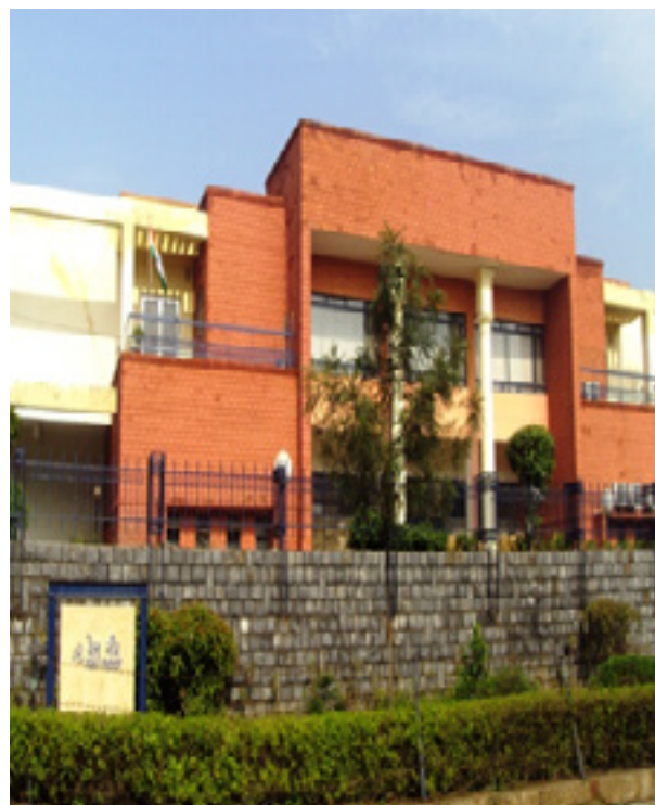
Railneer Plant Nangloi
