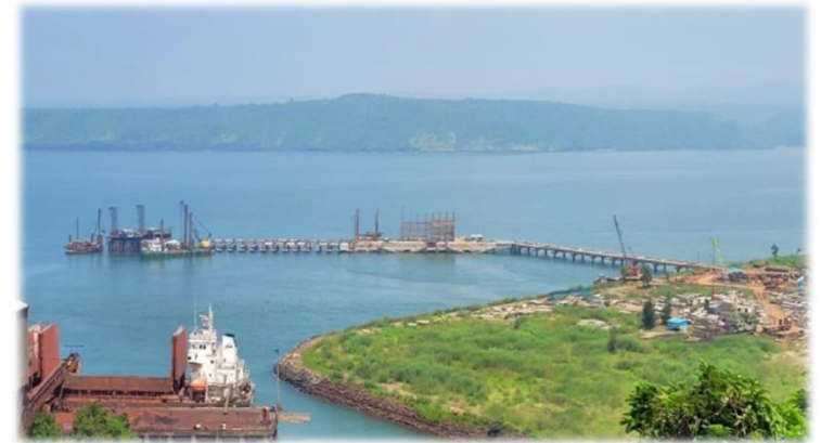
LPG construction at Jaigarh Port
