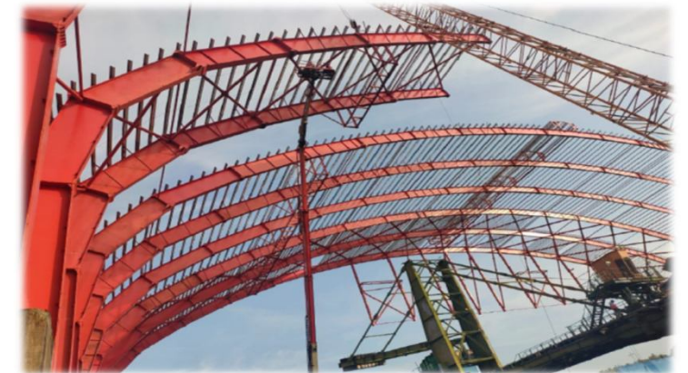
Work on Cover shed at South West Port, Goa
