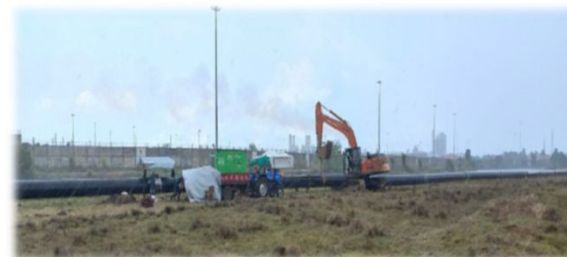
Setting up slurry pipeline
