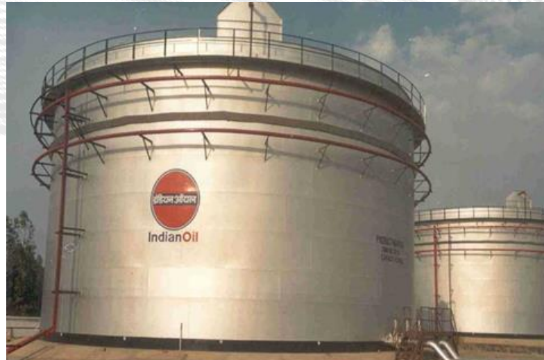
Cone / Dome Roof Tanks
