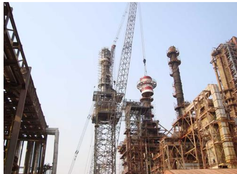
Maintenance, Shut Down / Revamp
