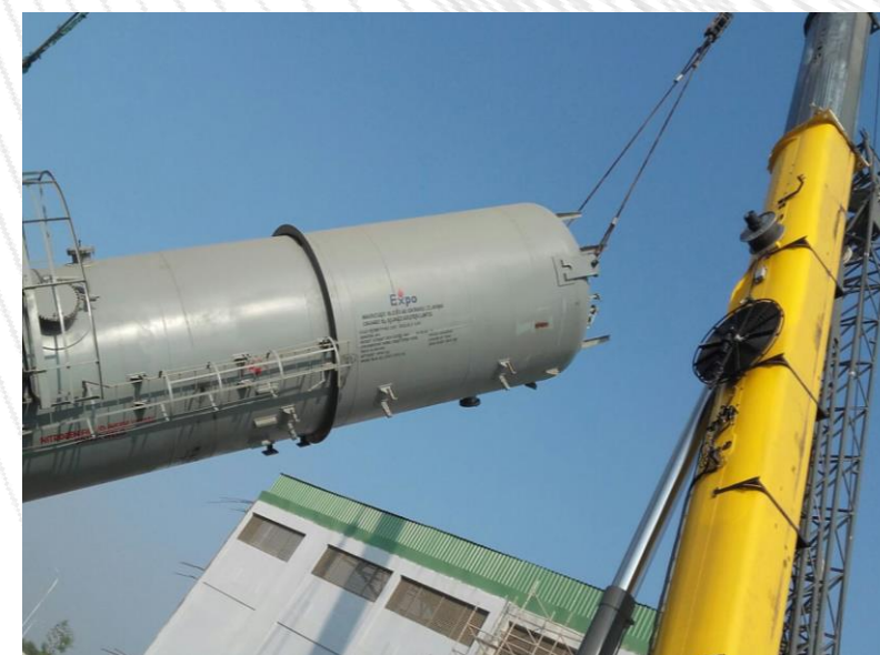
Fabrication & Erection of Equipments
