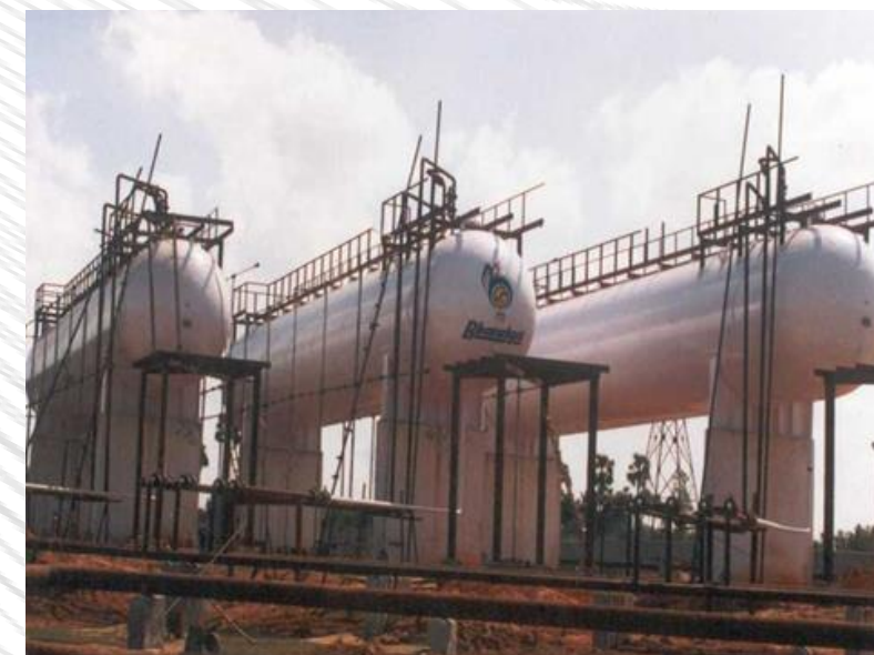
Bullets – Mounded Storage & Above Ground Bullets
