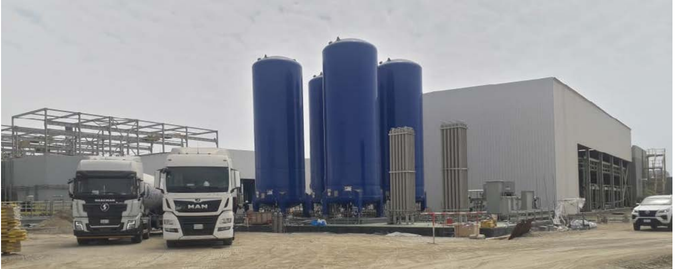
Customer installation of 4 x 80KL LCO 2 Tanks at Saudi Arabia
