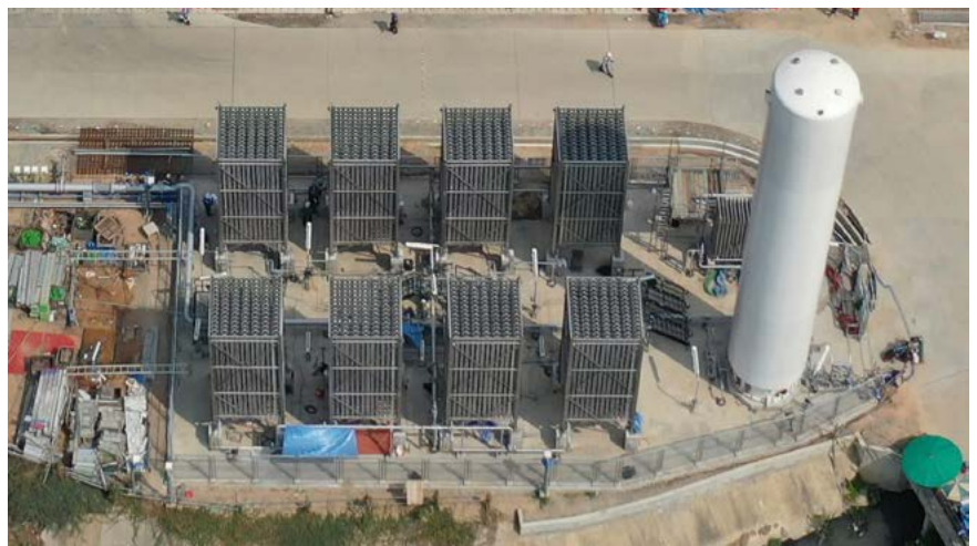
Installation of complete N2 package at Thailand 150kl + 8 vaporisers
