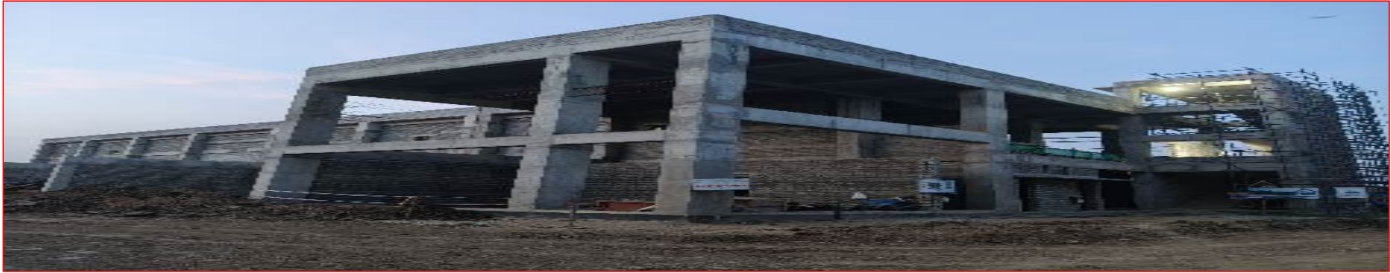
CONTROL ROOM BUILDING
