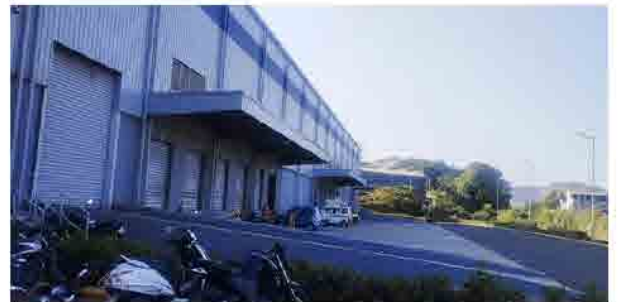
Building No B200, Shed 200, Indran Logi Indospace Industrial & Logistics, Ajivali, Khalapur Raigad - Khopoli
