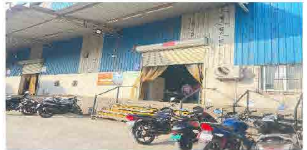
Santosh Warehousing Complex, Shil Phata Panvel Road, Dhansar Village, Taloja, Navi Mumbai
