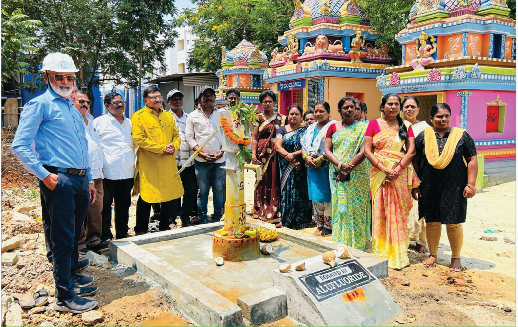
Installed Borewell at Mulagada, Visakhapatnam for the Development of Community Infrastructure.
