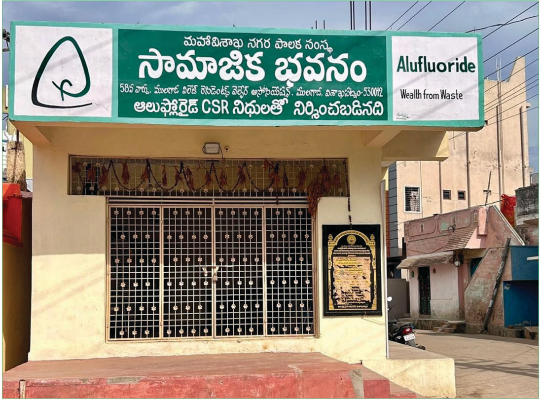
Constructed Community Hall at Mulagaga, Visakhapatnam for the Development of Community Infrastructure.
