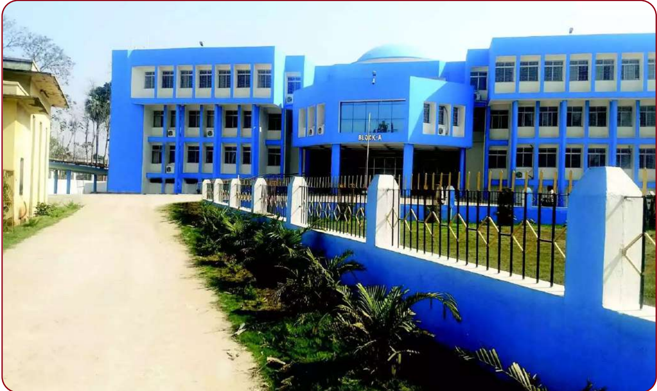
Collectorate Building Daltonganj, Jharkhand
