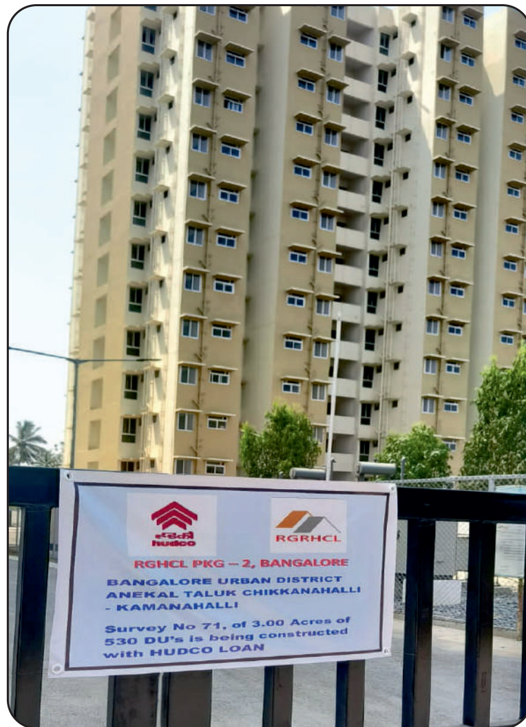
EWS Multistorey housing programme Bengaluru, Karnataka
