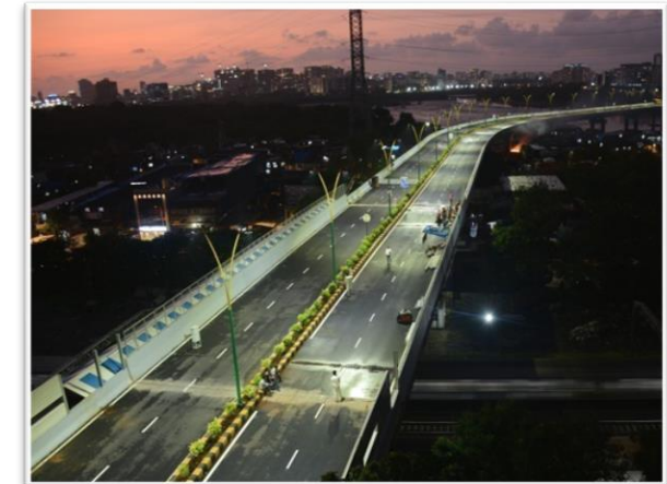
BKC- Chunabhathi Flyover
