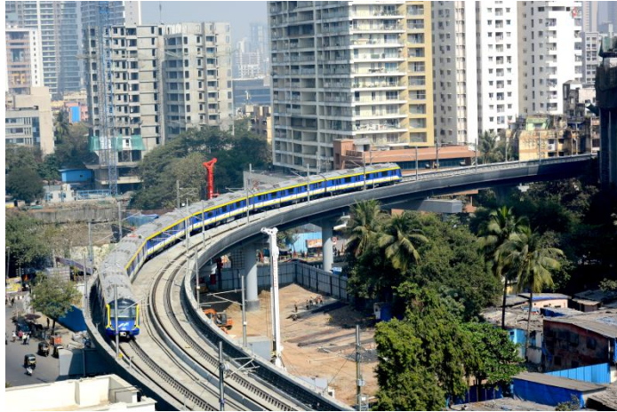
Mumbai Metro Line 2A
