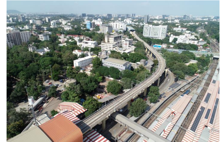
Pune Elevated Metro
