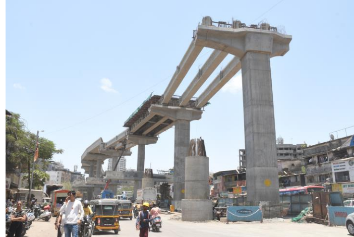
Mumbai Metro Line 9
