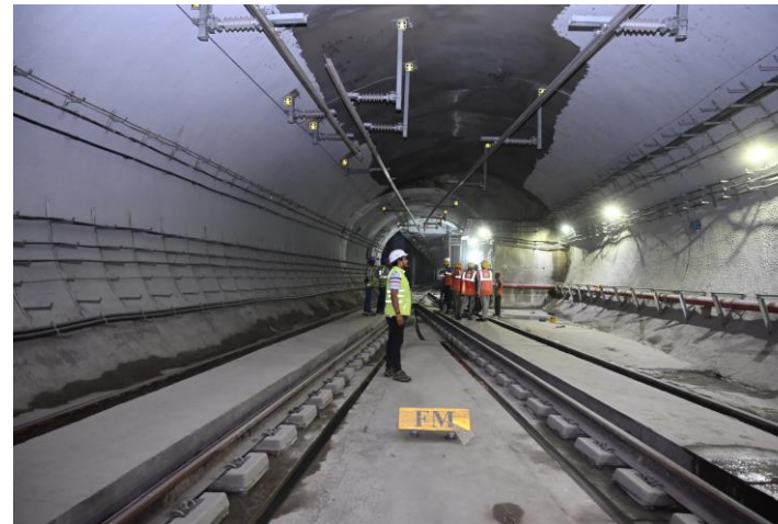
Mumbai Metro Line 7A
