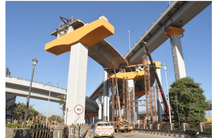
Sewri Worli Elevated
