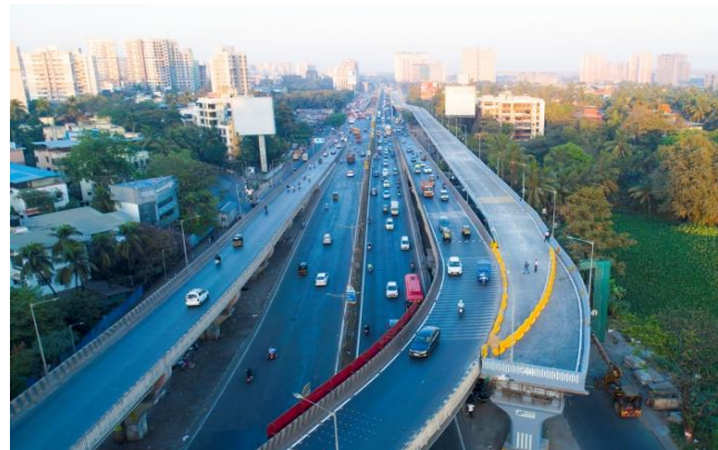
Chheda Nagar Flyover Part 1
