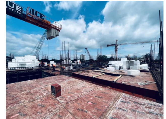
Pune Underground Metro
