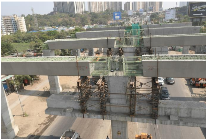
Mumbai Metro Line 4A
