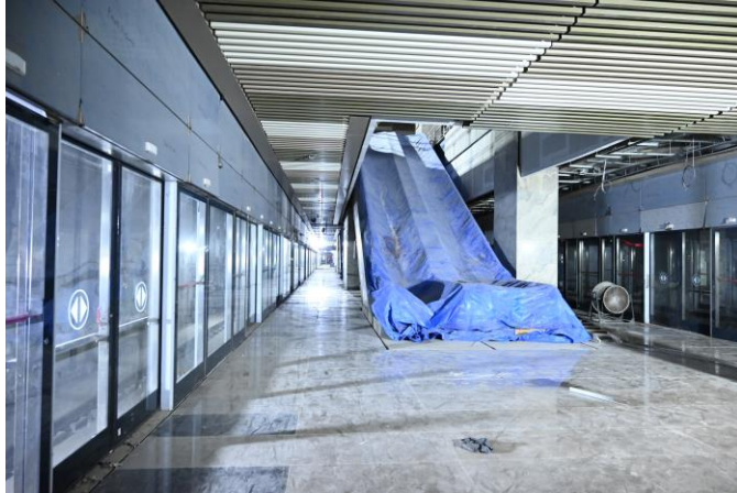
Mumbai Underground Metro Line 3
