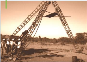
Conventional drill rig
