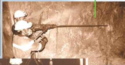
Drilling by hand-held hammer
