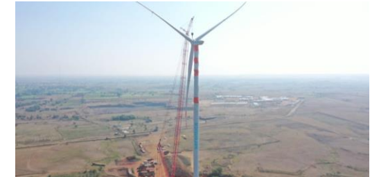
1st wind turbine installed
