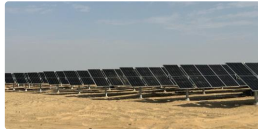
Modules installed at site
