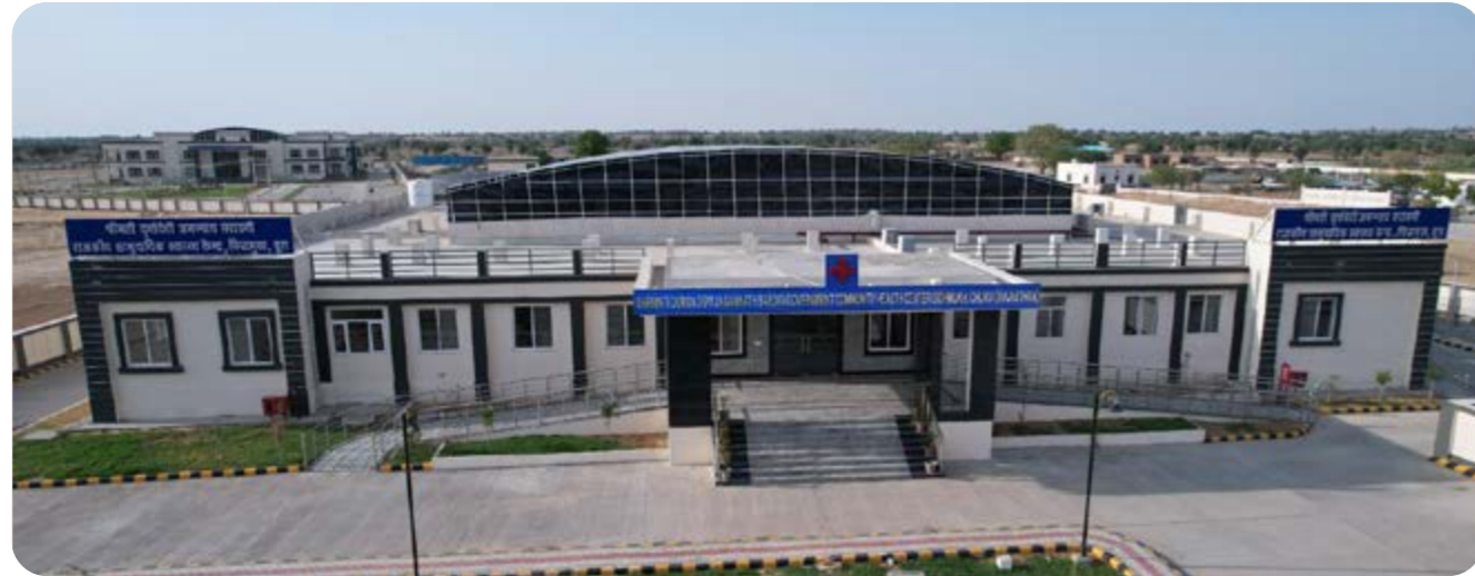
Construction of Smt. Durga Devi Jagannath Sarogi Government Community Health Center, Sidhmukh, Churu, Rajasthan
