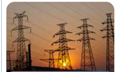
Transmission system in Rajgarh II (BOOT)
