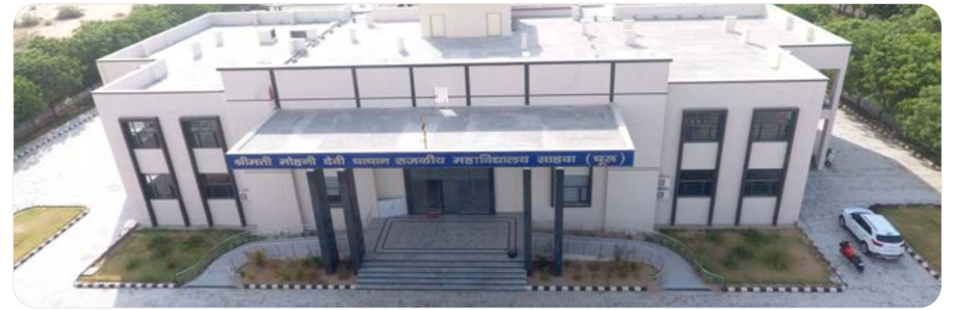
Construction of Smt. Mohini Devi Chachan Government College, Sahawa, Churu, Rajasthan
