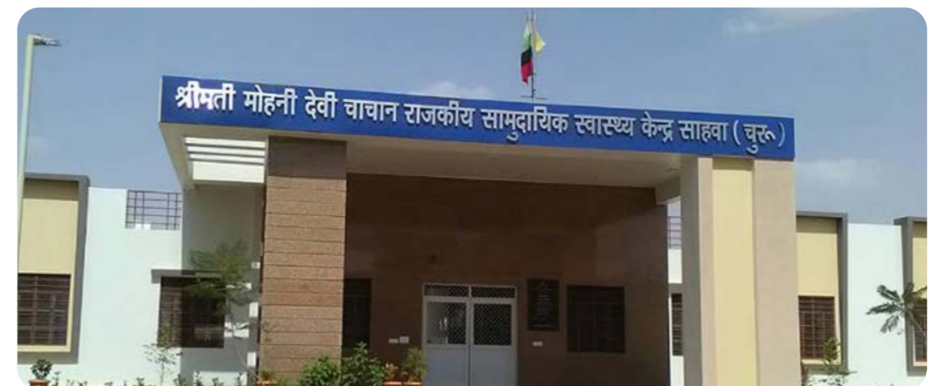
Construction and maintenance of Smt. Mohini Devi Chachan Rajkiya Samudayik Kendra, Sahawa, Churu, Rajasthan
