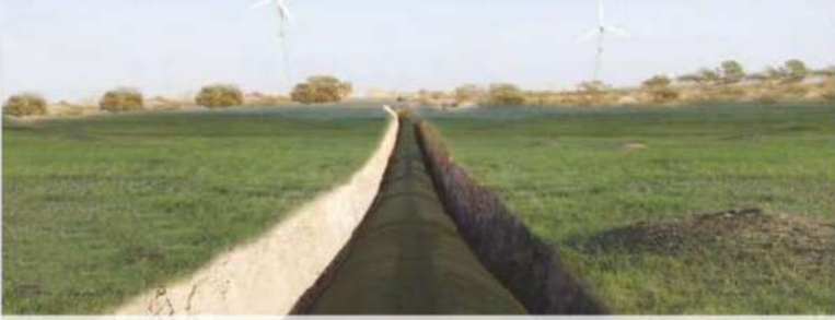
3000 MM Dia MS Pipeline, Sauni Yojana, Gujarat
