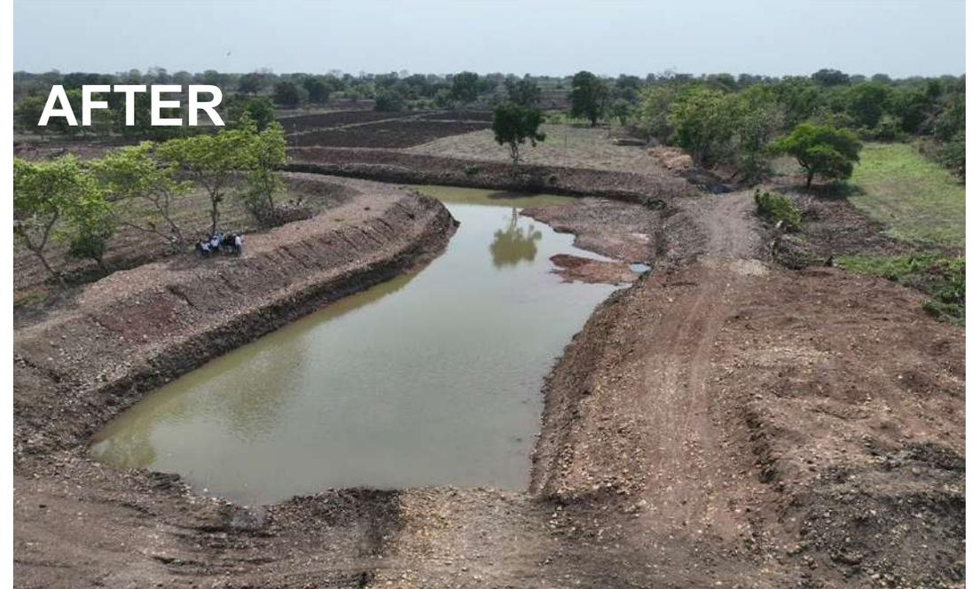
Together with NAAM Foundation we created a 4km water canal to avoid flooding of neighboring crops and to conserve and direct water towards ponds and wells for sustained utilization. This will enable farmers in three villages (Ambala, Bhingi, Warang) to grow a second crop and increase the livelihoods of their families and communities.
