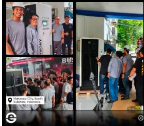
Heavy-duty DC charger installation in Indonesia
