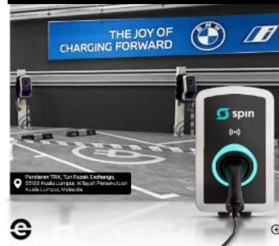
AC charger installation at BMW Malaysia
