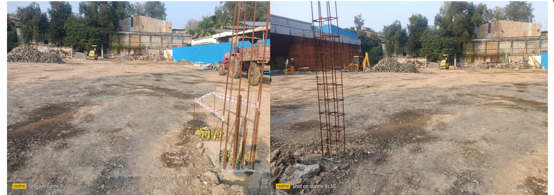
Extension of existing plant to cater to EV OEM
