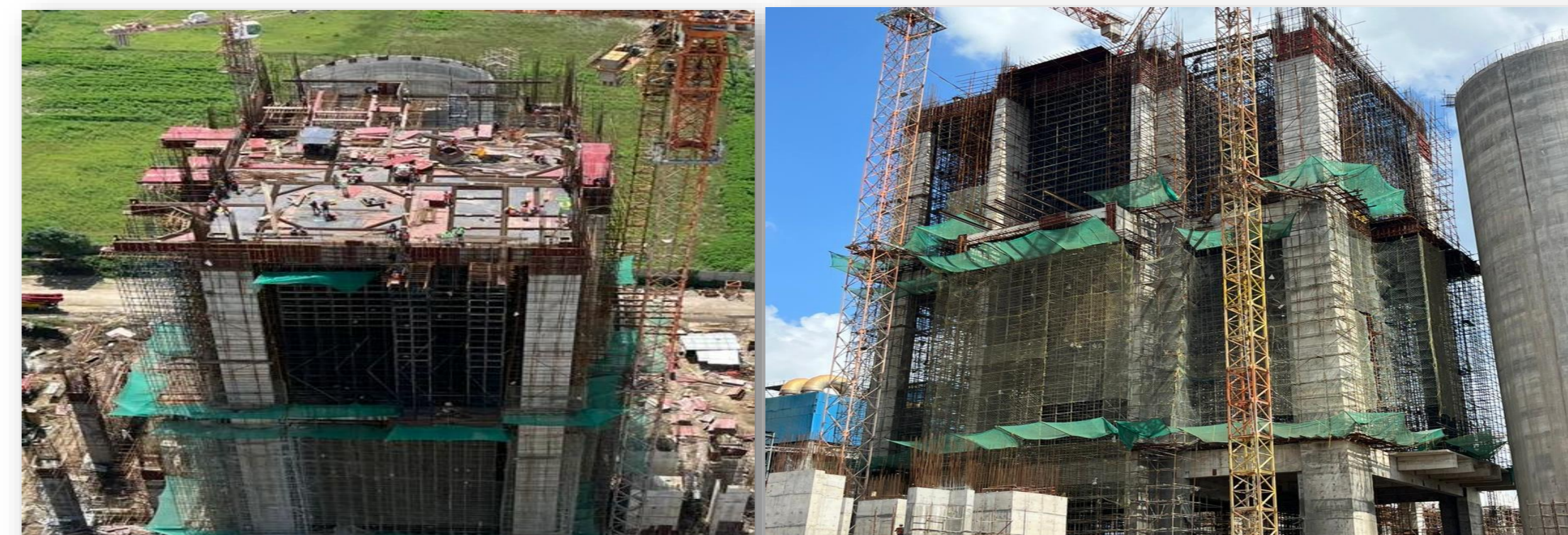
Preheater Building-Panna Line-II
