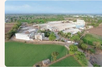
AGL Idar Plant (Floor Tiles)
