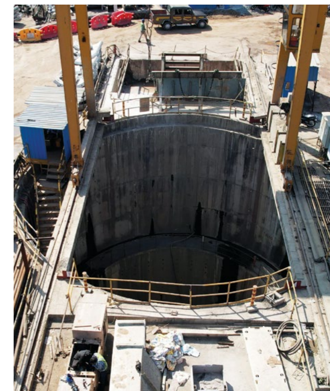
▶ TBM launch shaft with 12 metre diameter, Dharavi Wastewater Treatment Facility
