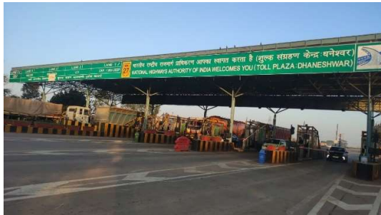
Dhaneshwar Toll Plaza
