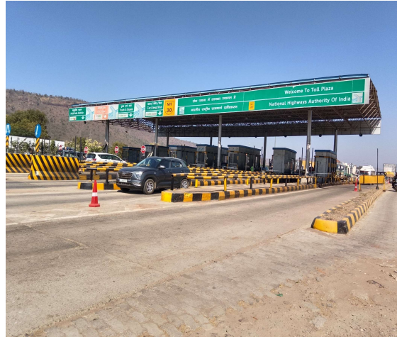
Kherwasani Toll Plaza
