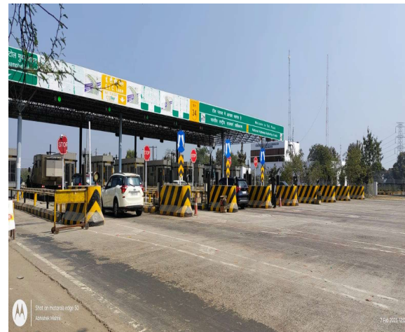
Boharipar Toll Plaza
