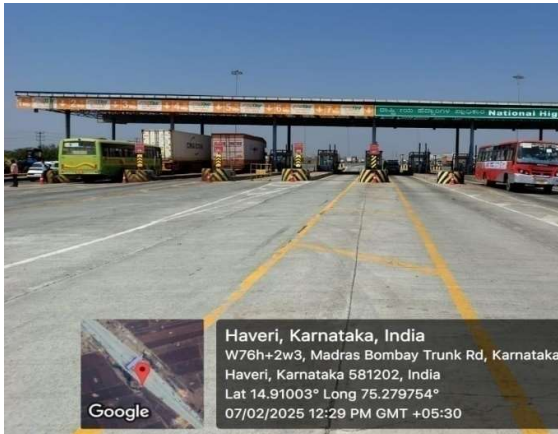
Bankapur Toll Plaza
