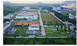
Unit-2, Atchutapuram 10Bn units, 161 KL
