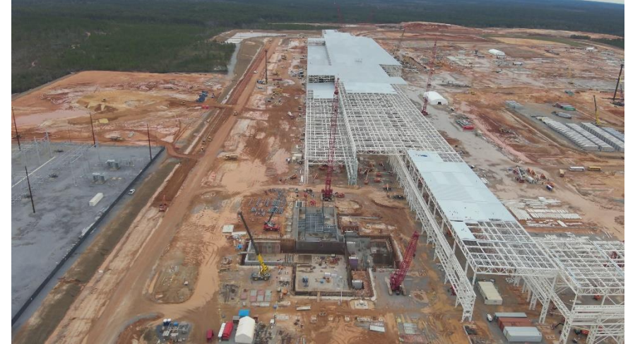
Bay Minette site and construction, January 15, 2025
