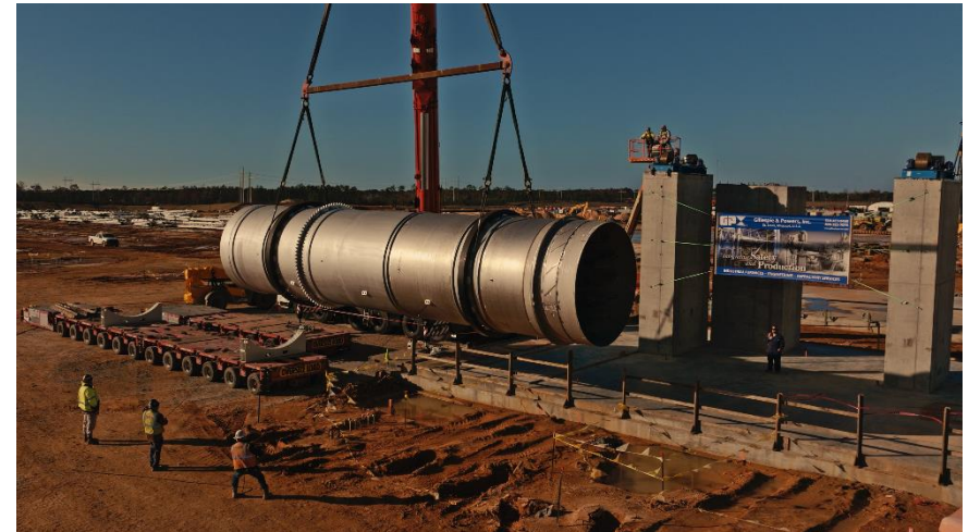
Recycle/remelt center kiln installation
