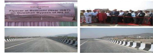
Construction of 2 lane flyover on Guwahati Bypass of NH-115 (earlier NH-37) in the state of Assam
