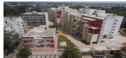
Construction of 92 flats at Mahadev Towers, Bhopal for MP Housing & Infrastructure Development Board
