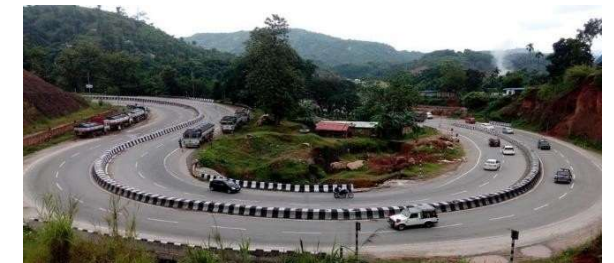
Widening & Strengthening of existing National Highway from 2 lane to 4 lane of Sonapur to Guwahati section of NH-115 (earlier NH 37)
