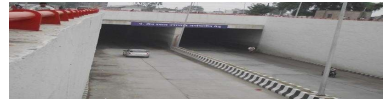
Construction of RUB at Badli, New Delhi
