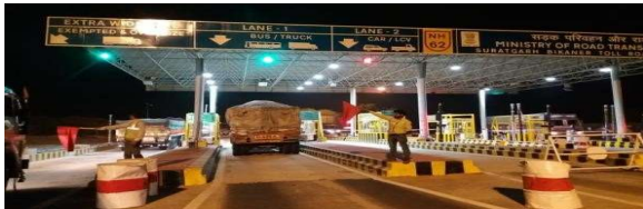
Development & Operation of Bikaner- Suratgarh Section of NH-62 (earlier NH-15) in the state of Rajasthan
