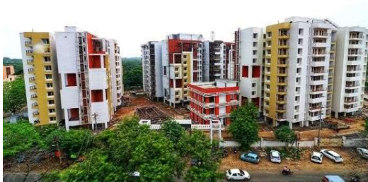
Construction of 222 Flats at Keelandev Tower, Bhopal for MP Housing & Infrastructure Development Board
