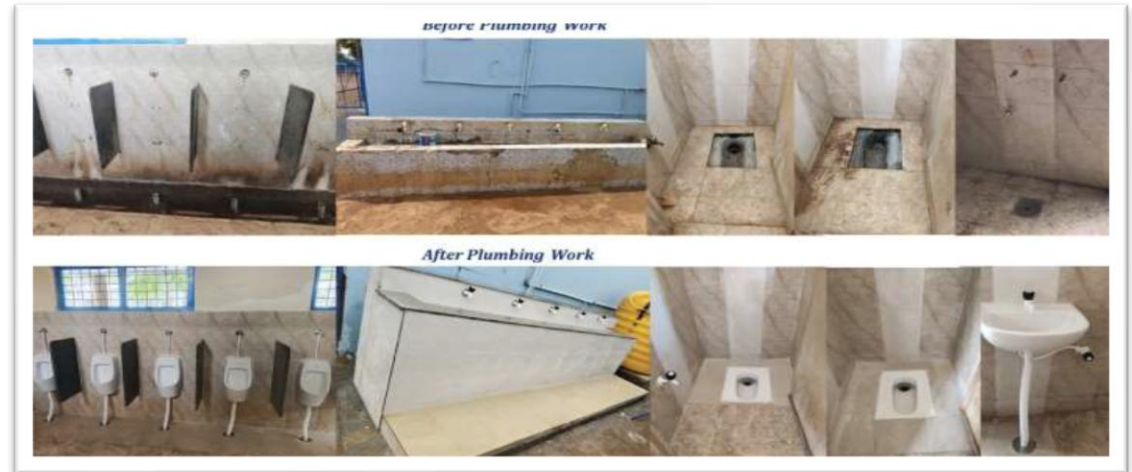
5S Plumbing Renovation Work At Ghps Hennagara
